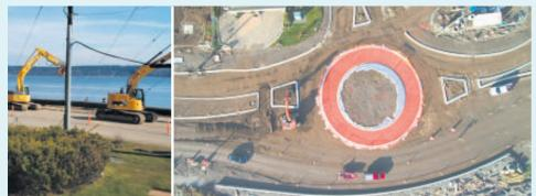
Construction continued on major upgrades to water, sewer and storm drains north from Rockland Road to 1st Avenue. Above-ground improvements from Rockland Road to the Big Rock boat ramp are scheduled for early 2021 and include burying overhead wires and installing a roundabout centre feature inspired by tidal pools.
