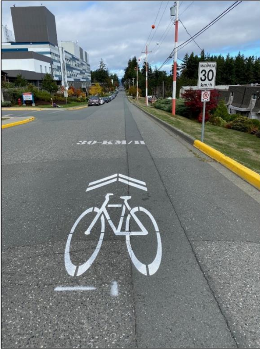
New 30 km/hr signage and sharrow pavement marking on Birch Street, northbound, north of Evergreen Road (by the hospital). Photo by City of Campbell River
