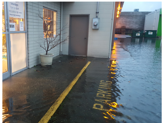
Figure 9. Flooding downtown during the January 2018 king tide. High ocean water levels prevent water from flowing into the sea through storm drains.
