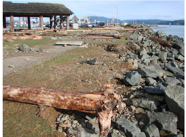
Figure 8. Damage to Ostler park after the March 12, 2012 storm, where winds gusted up to 137 km/hr.
