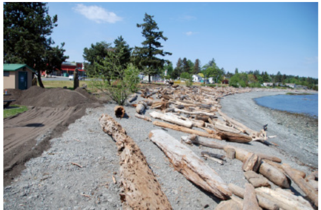
Figure 12. Rock armouring damaged by powerful waves at Osler Park during the March 12, 2012 storm (top) and soft shore restoration work that will provide natural shoreline protection, being implemented at Adams Park (bottom).
