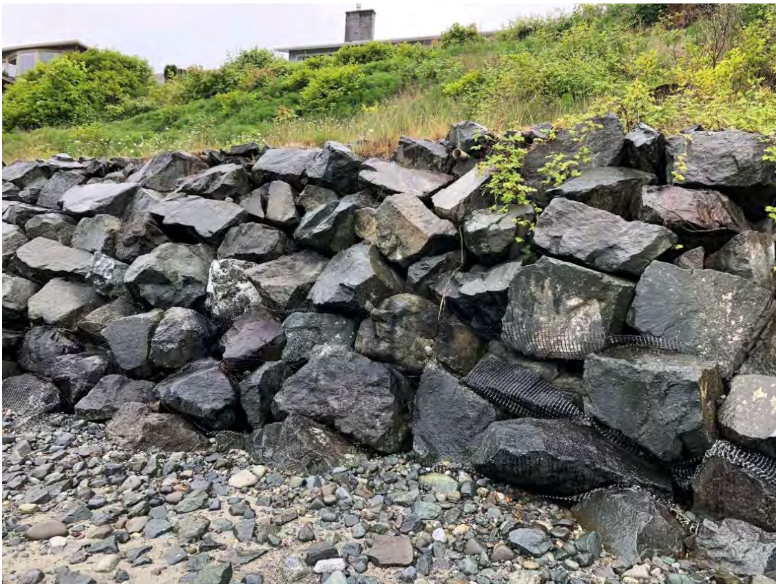
P14: Loosely stacked boulder seawall near 4635 Discovery Dr.
