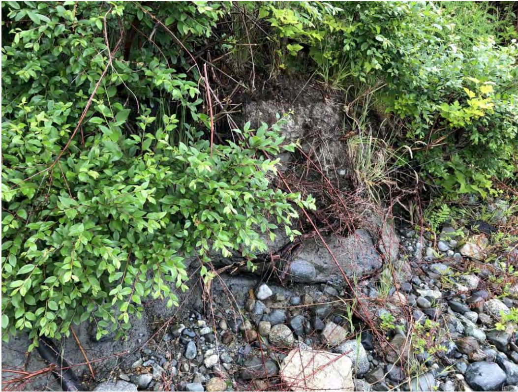
P24: Toe erosion near 4535 Discovery Dr.
