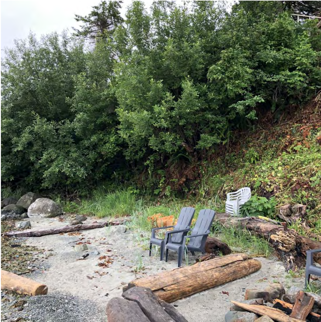
P47: Toe erosion near 4315 Discovery Dr.
