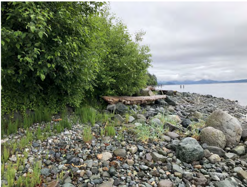
P27: Toe erosion near 4535 Discovery Dr.
