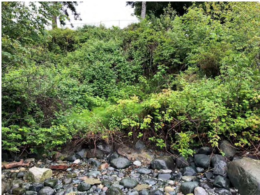
P12: Toe erosion near 4655 Discovery Dr.
