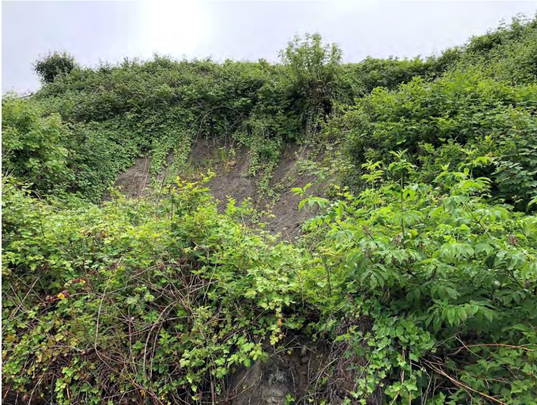
P17: Substantial erosional scarp near 4565 Discovery Dr.
