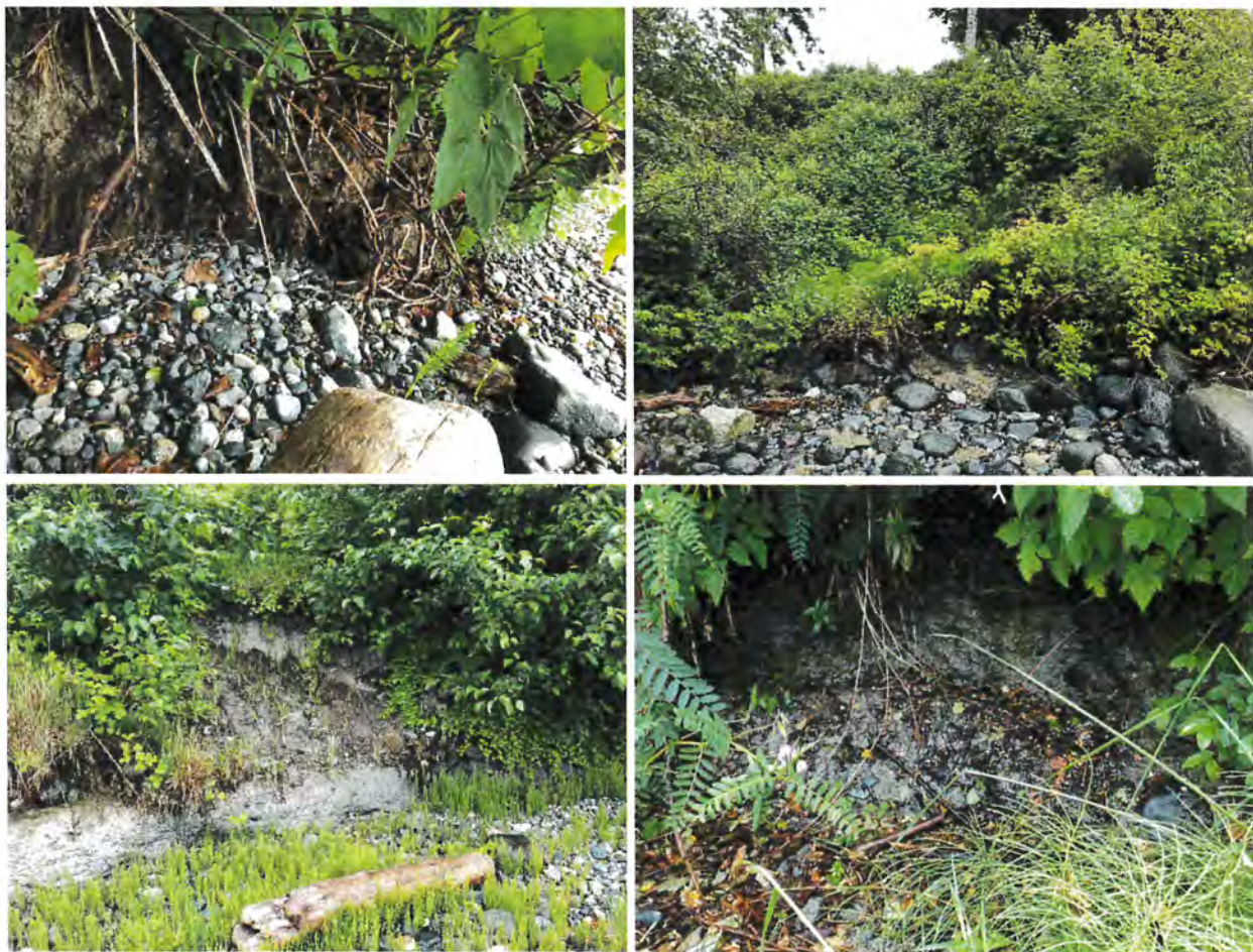
Photos 1, 2, 3, 4 – This set of photos shows general examples of toe erosion of the foreshore slope.
