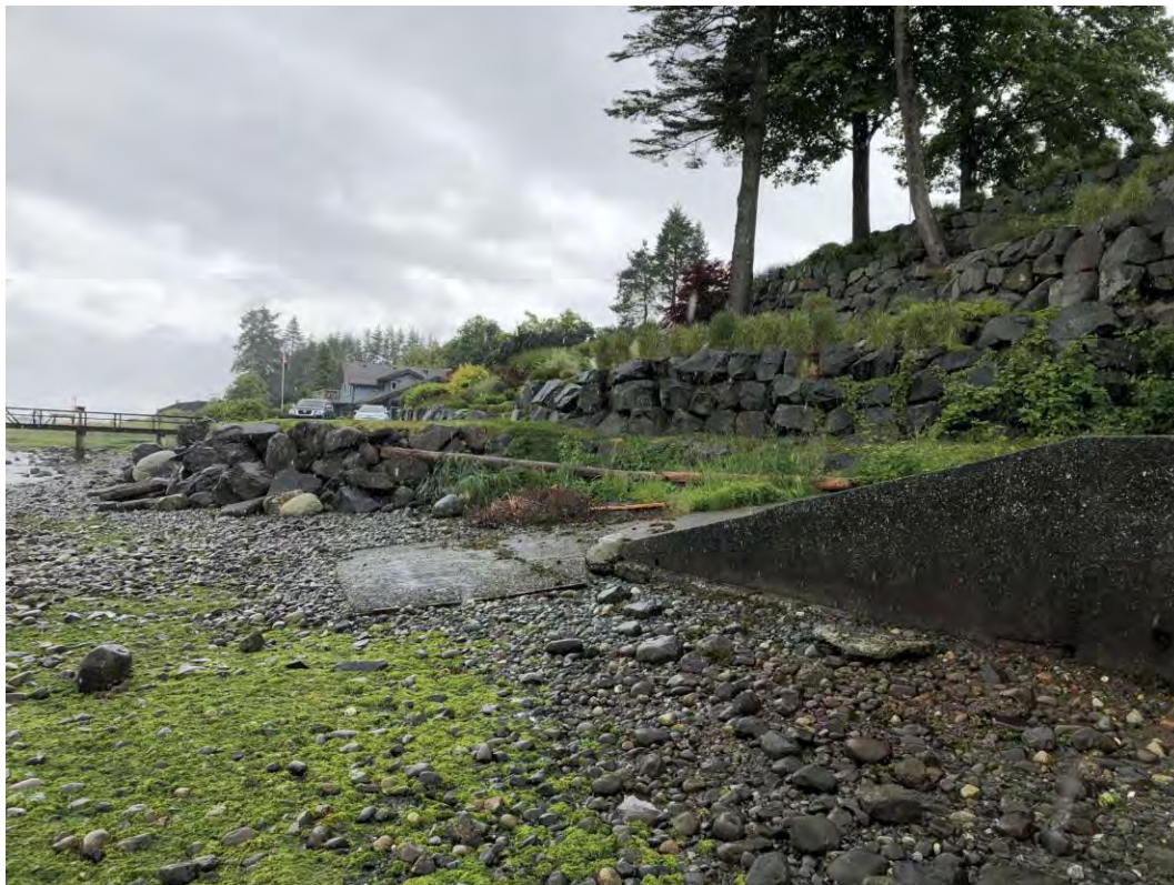
P61: Tiered slope and boulder stack walls near 3847 McDougall Way
