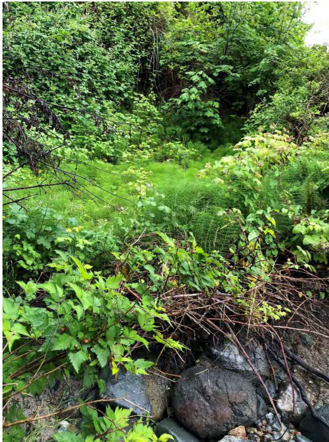
P10: Substantial erosional scarp obscured by common horsetail vegetation near 4655 Discovery Dr.
