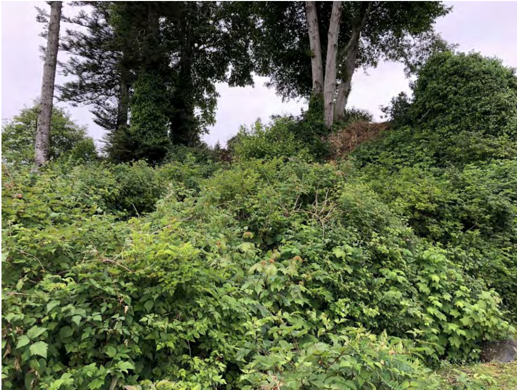
P42: Crest erosion near 1800 Hughes Dr.
