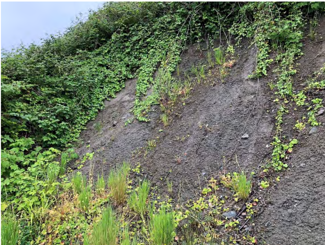
P18: Substantial erosional scarp near 4565 Discovery Dr.
