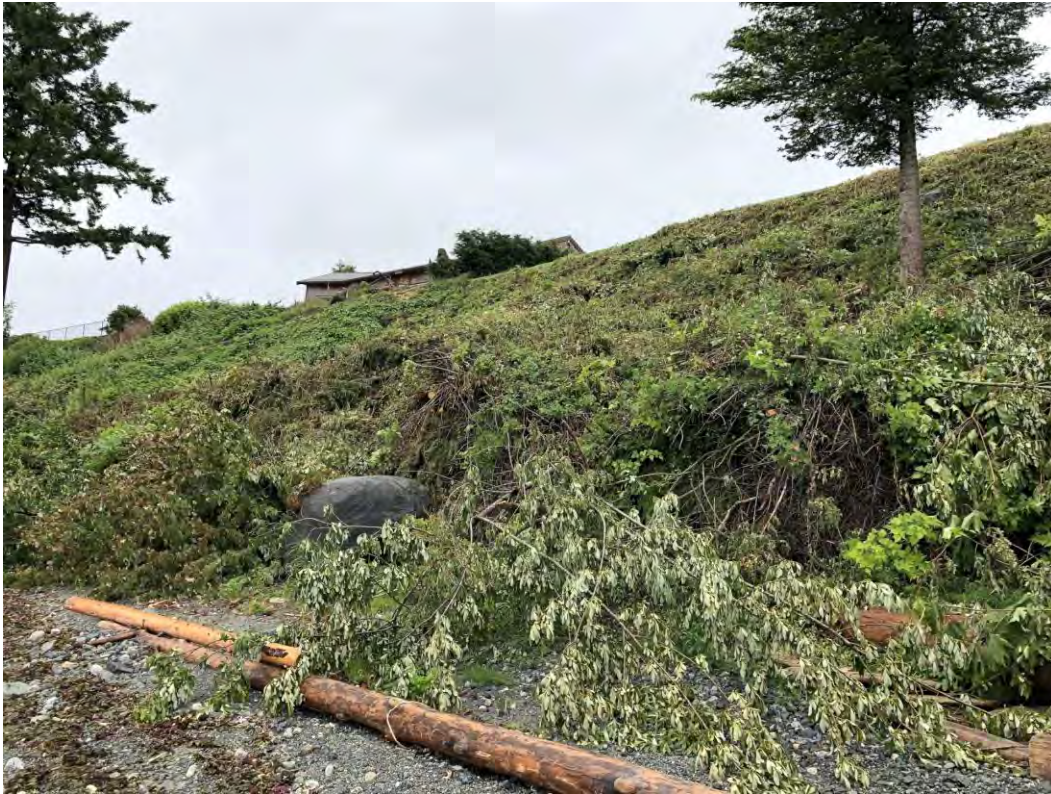
P56: Toe erosion near 4065 Discovery Dr.
