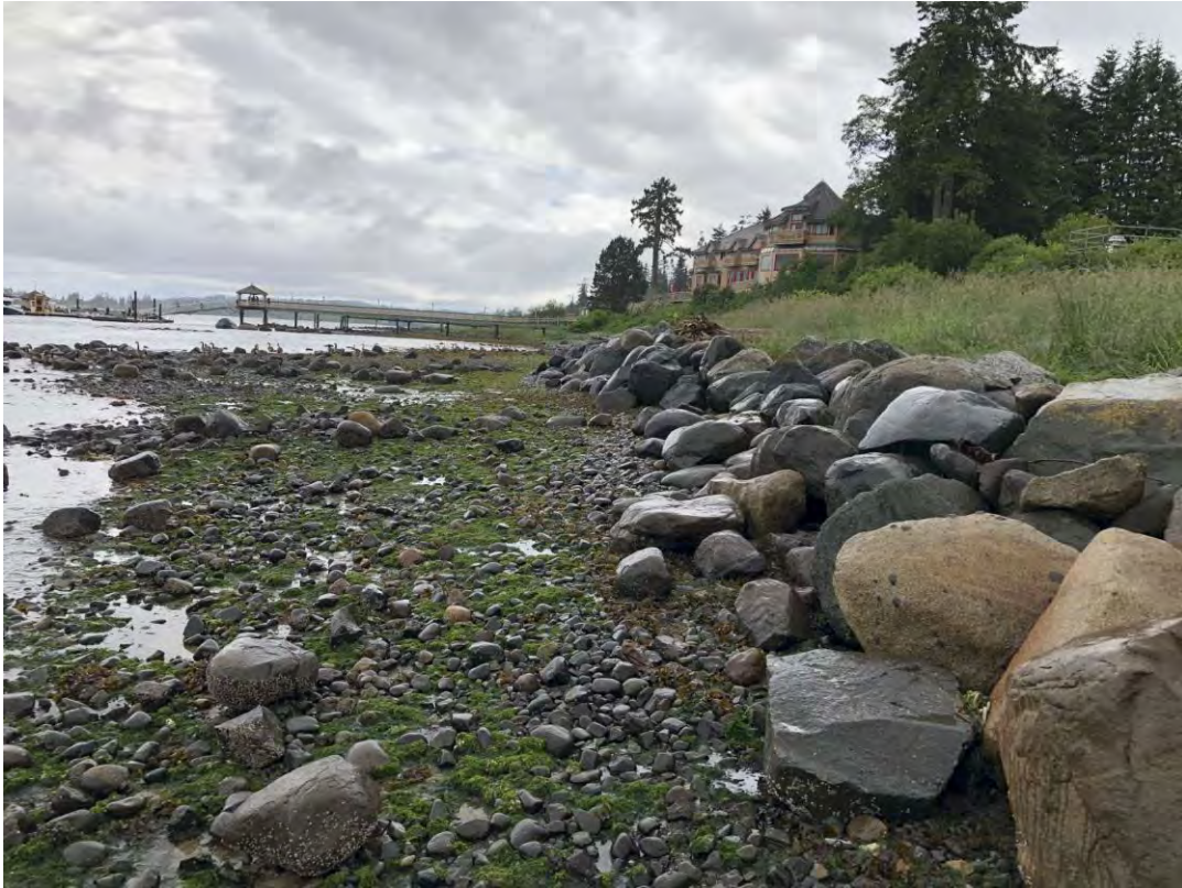
P64: Loosely stacked boulder seawall near 3817 McDougall Way
