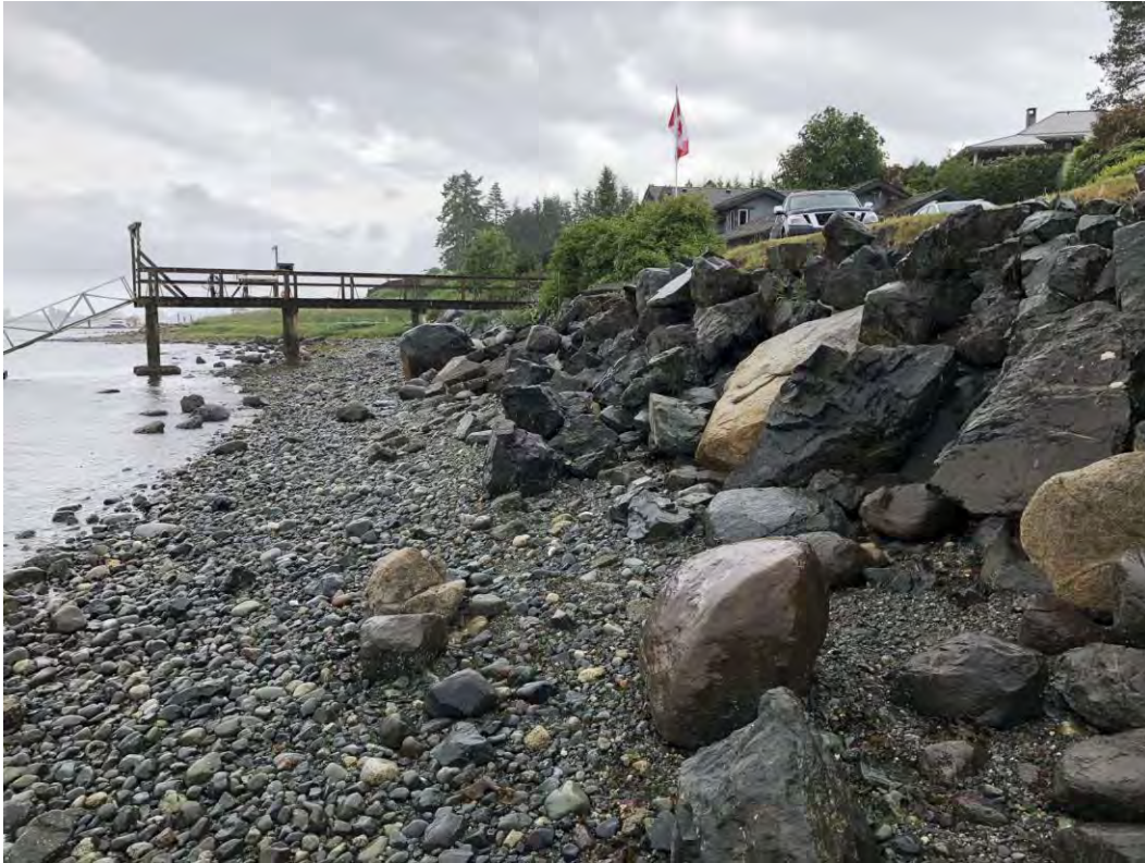
P62: Loosely stacked boulder seawall near 3847 McDougall Way
