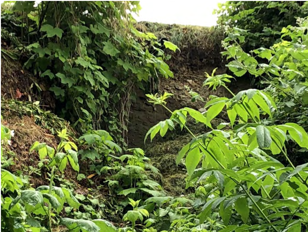
P45: Close up of crest erosion near 4365 Discovery Dr.
