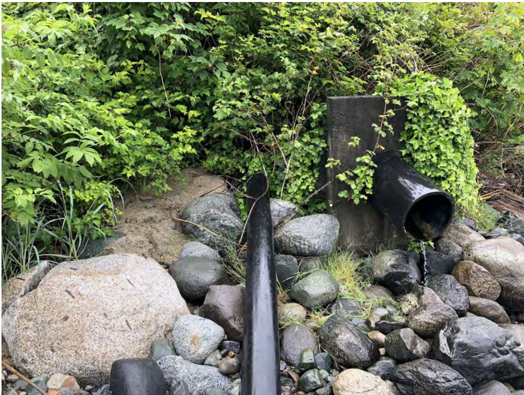
P16: Drainage pipes discharging at toe near 4575 Discovery Dr.
