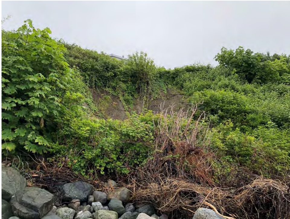
P19: Substantial erosional scarp near 4565 Discovery Dr.
