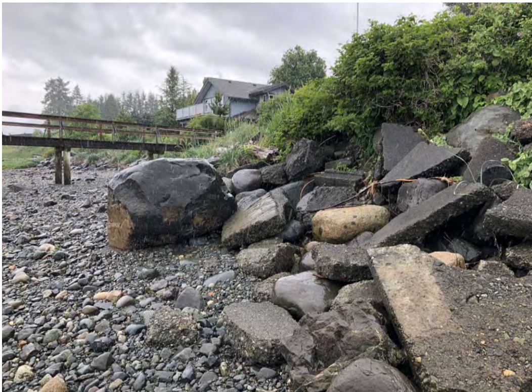
P63: Loosely stacked boulder seawall near 3847 McDougall Way
