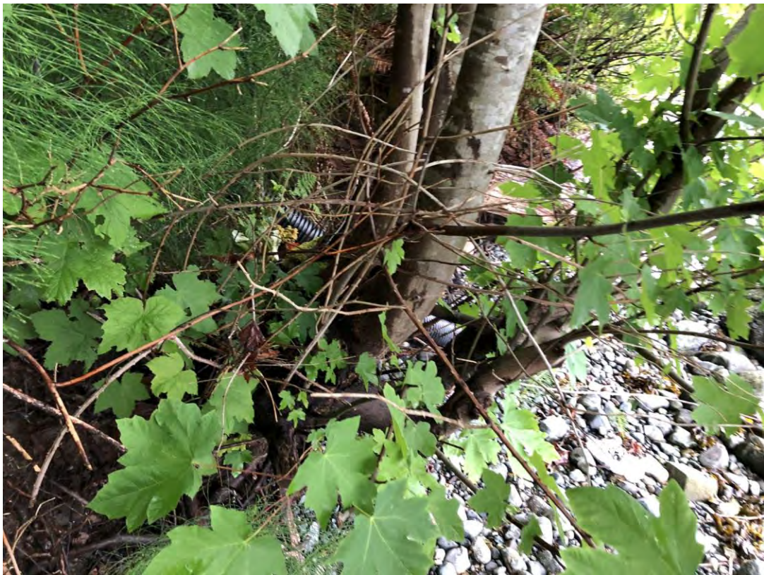
P08: Flexible drainage pipe near 4665 Discovery Dr.
