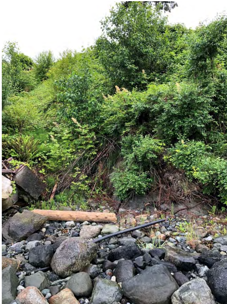
P22: Toe erosion near 4585 Discovery Dr.
