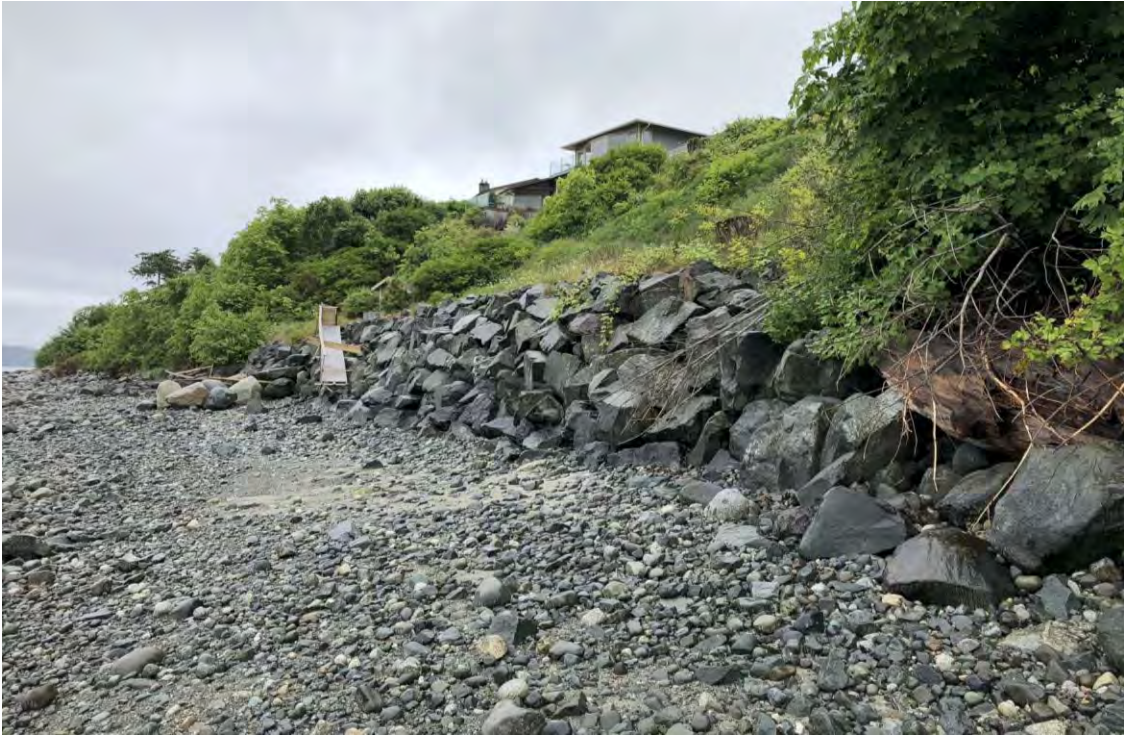
P13: Loosely stacked boulder seawall near 4635 Discovery Dr.
