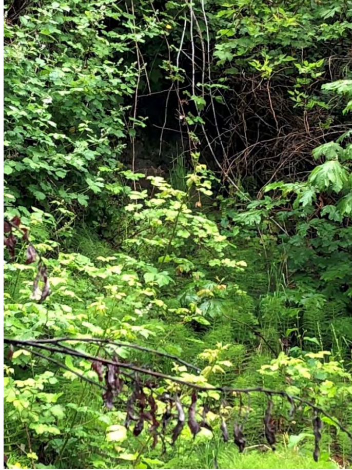
P11: Substantial erosional scarp obscured by common horsetail vegetation near 4655 Discovery Dr.
