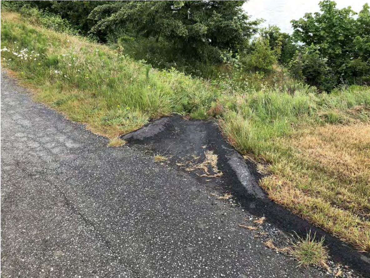
P66: Storm water discharge to crest of foreshore slope near 4730 Orange Point Rd.
