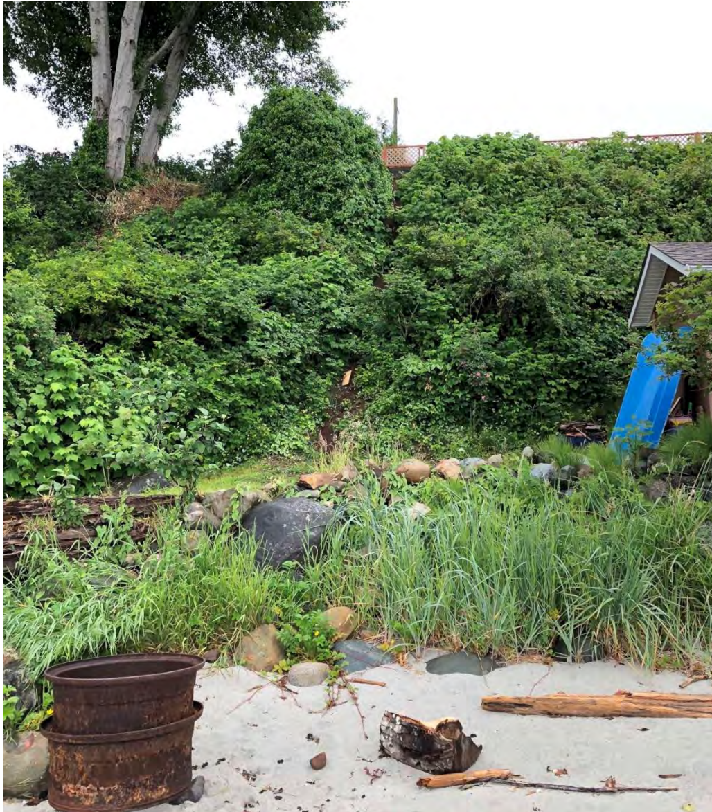
P41: Toe/crest erosion near 4385 Discovery Dr.
