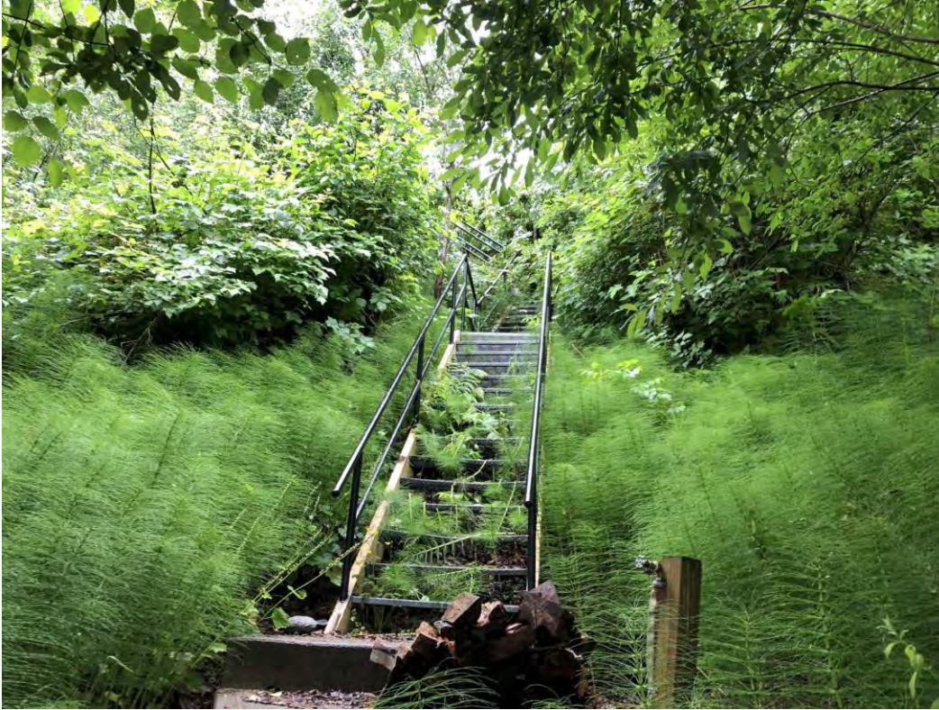
P05: Toe erosion obscured by common horsetail vegetation near 4665 Discovery Dr.
