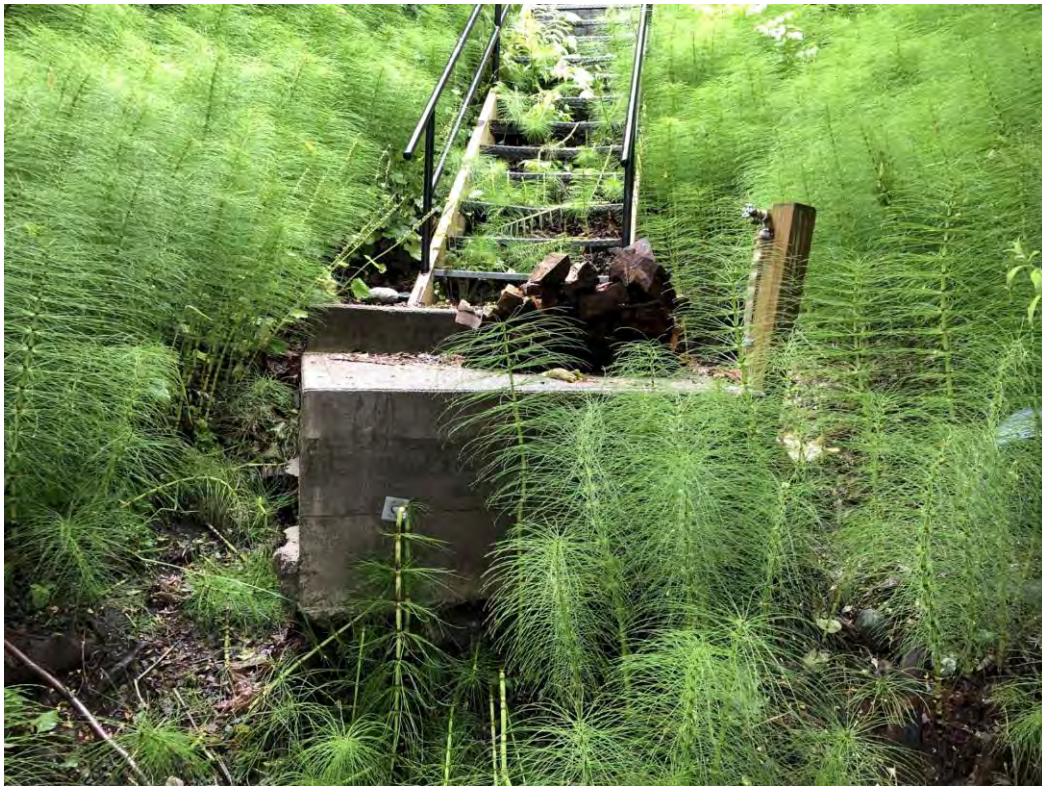
P06: Undermined concrete pad caused by toe erosion near 4665 Discovery Dr.
