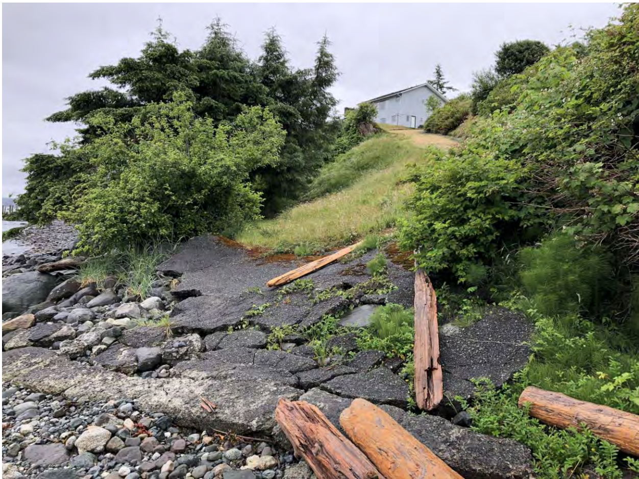
P01: Dilapidated boat ramp with toe erosion on both sides near 4785 Orange Point Rd.
