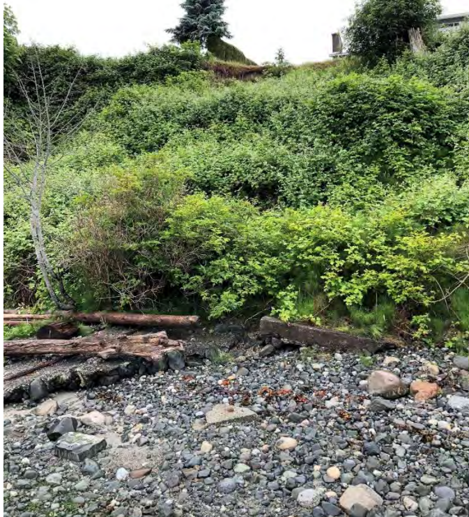
P03: Toe erosion and crest erosion near 4685 Discovery Dr.
