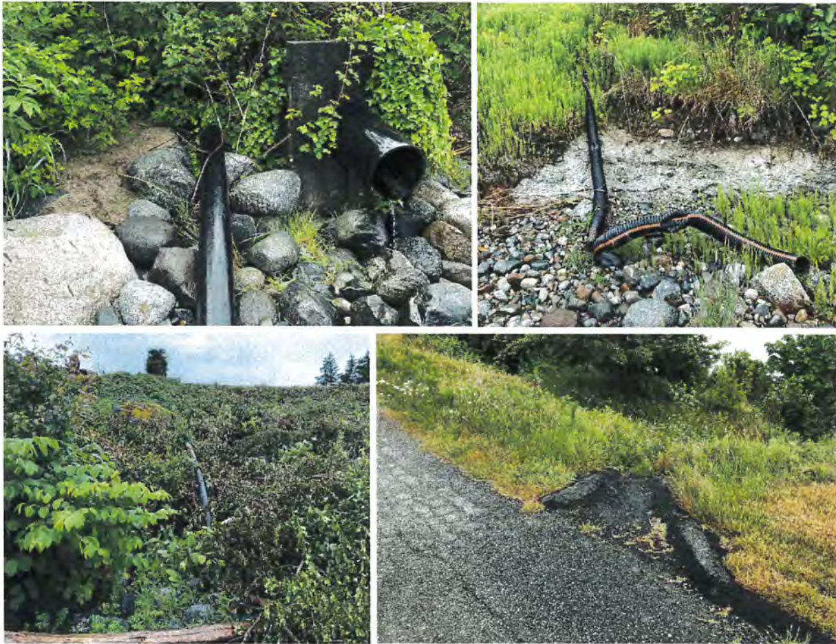
Photo 7 – Two drainage pipes discharging near the toe of the foreshore slope.
