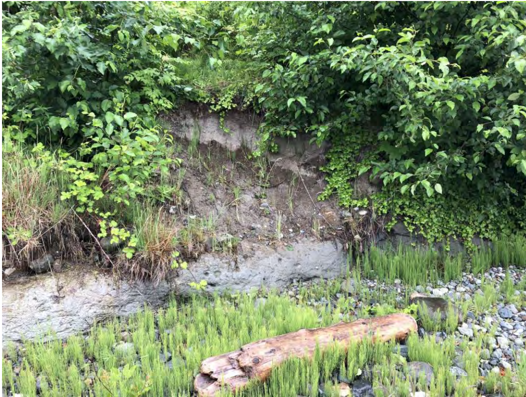
P26: Toe erosion near 4535 Discovery Dr.
