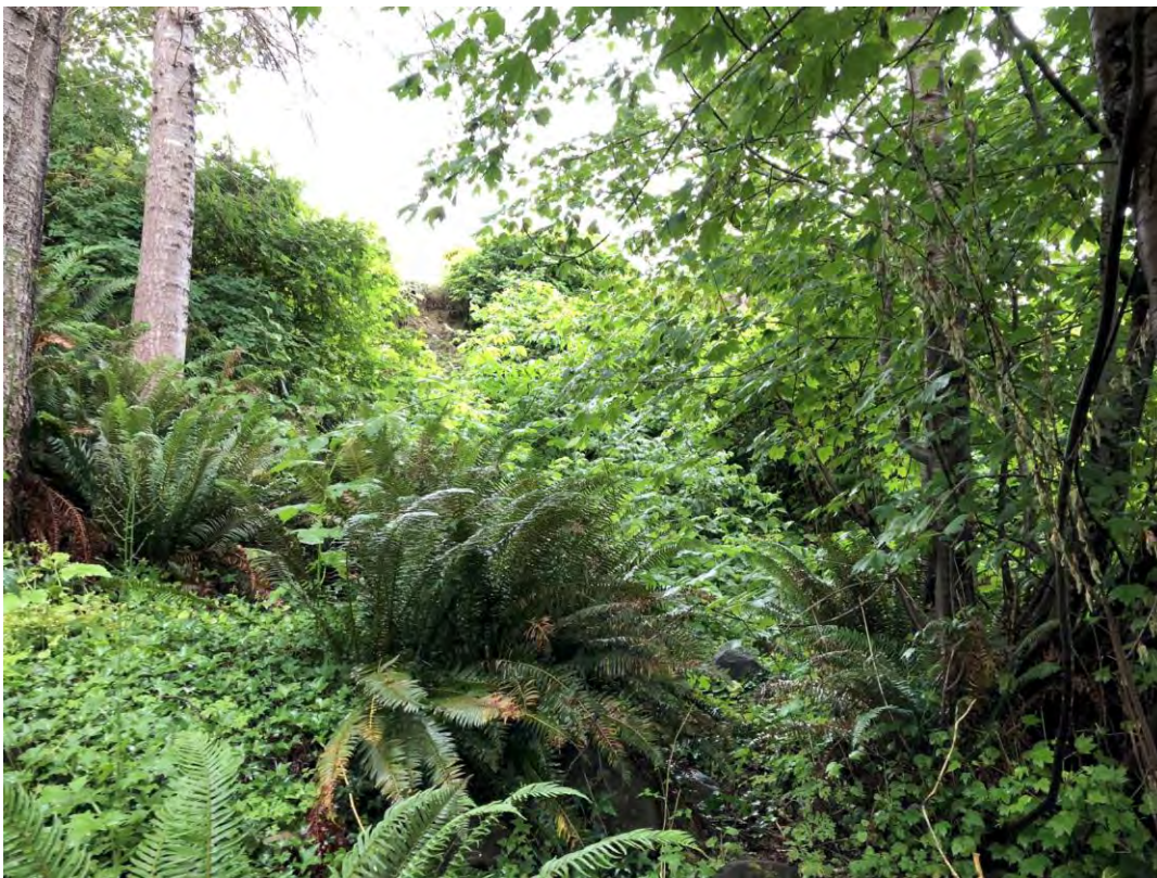
P43: Crest erosion near 4365 Discovery Dr.
