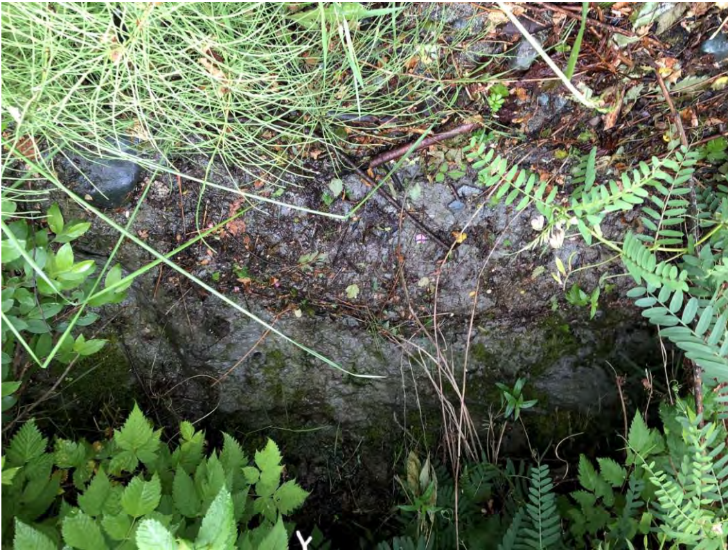
P57: Toe erosion near 4065 Discovery Dr.
