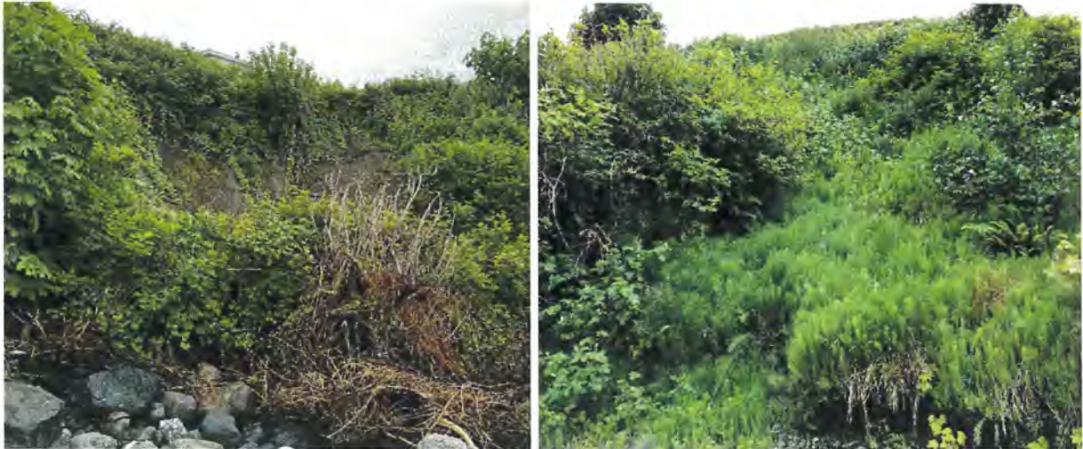
Photo 5 – Shows foreshore slope erosion at 4565 Discovery Drive.
