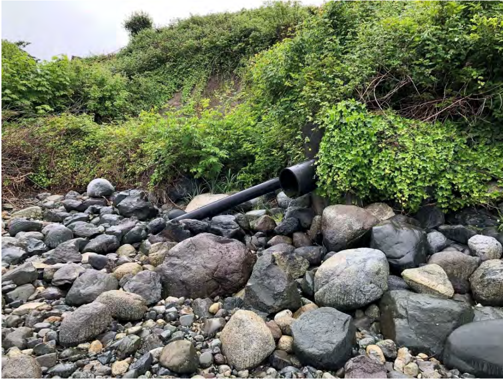
P15: Drainage pipes discharging at toe near 4575 Discovery Dr.
