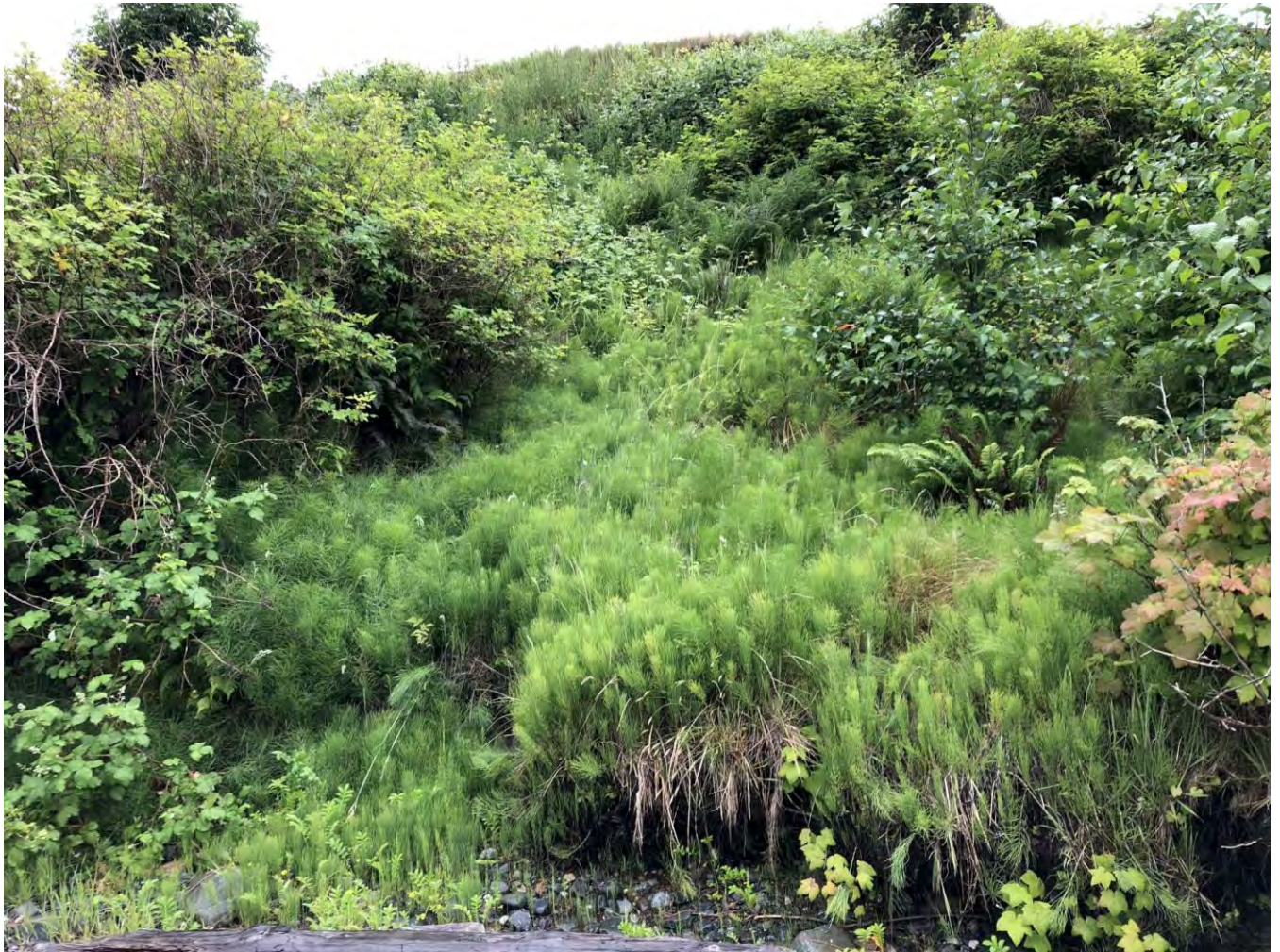
P02: Toe erosion covered with common horsetail vegetation near 4685 Discovery Dr.
