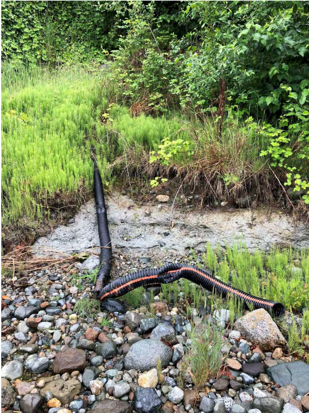
P25: Poorly installed drainage pipe and toe erosion near 4535 Discovery Dr.
