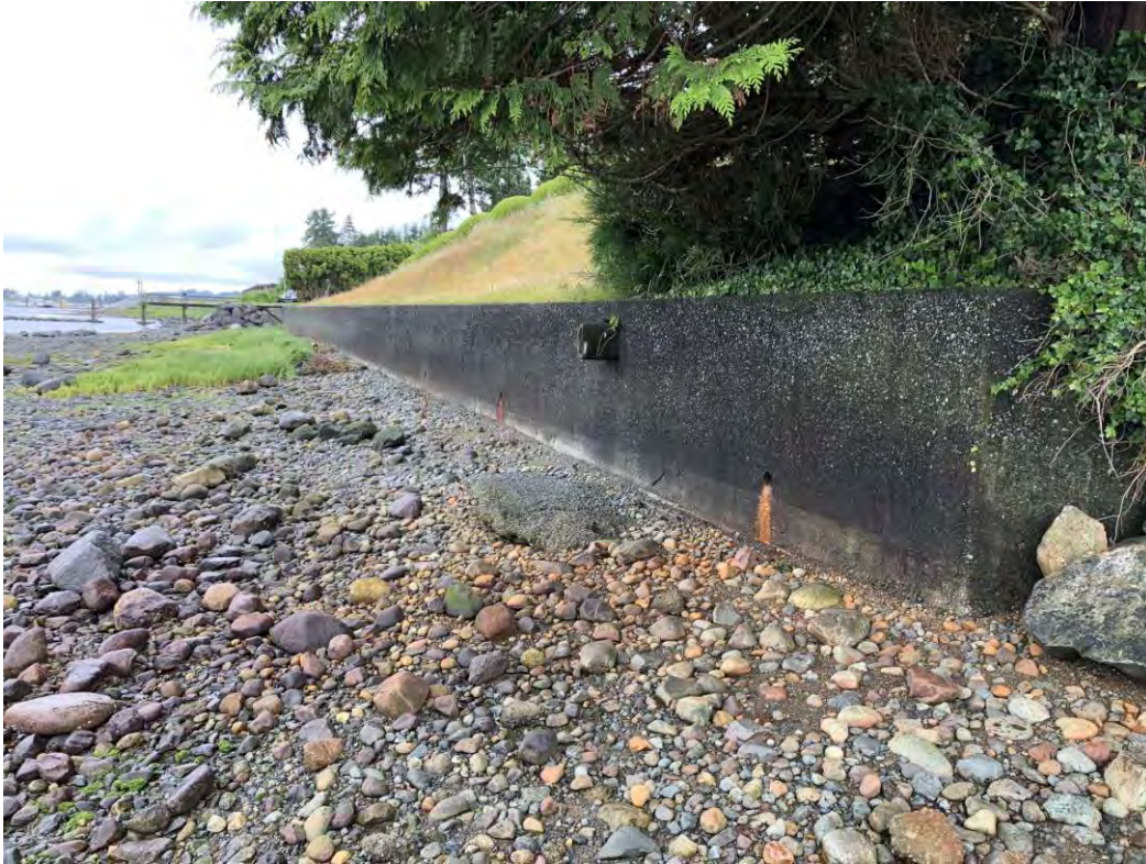
P60: Seawall near 3847 McDougall Way
