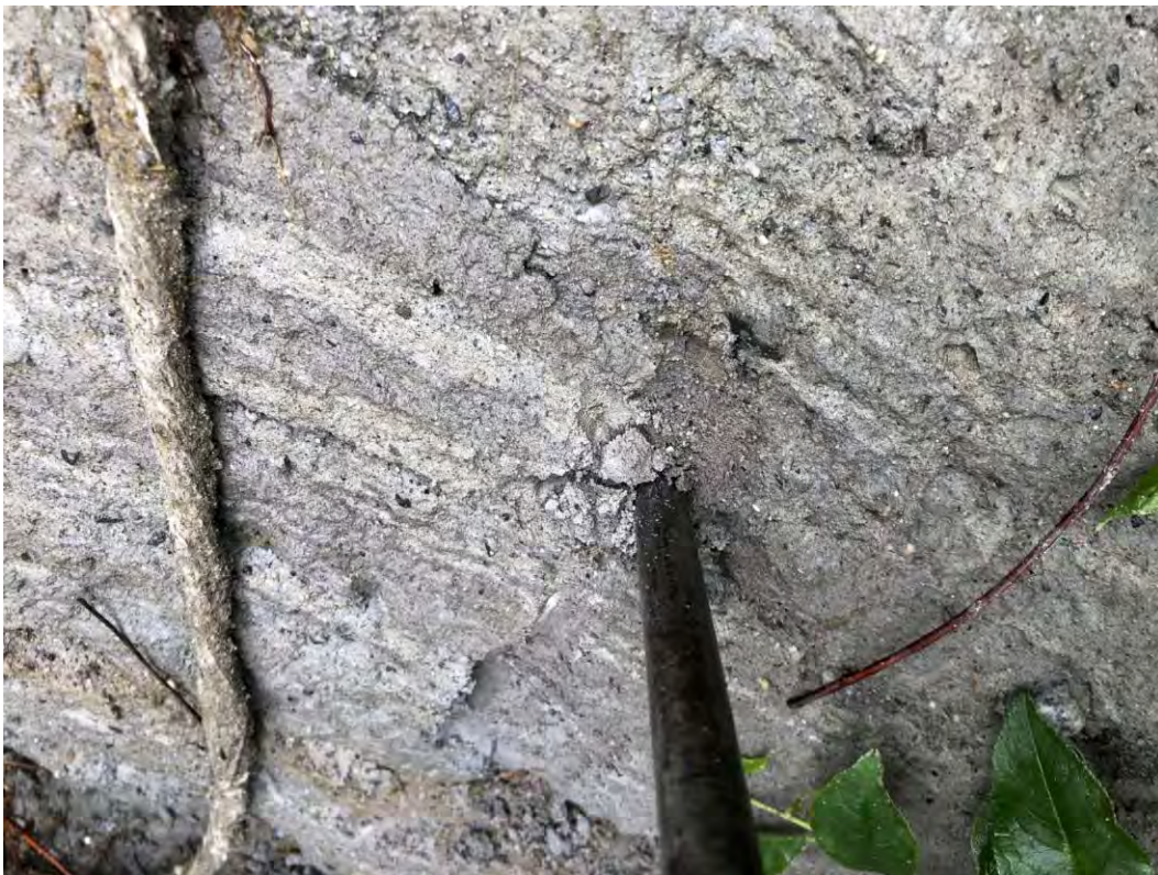
P24: Toe erosion exposing glacial till near 4535 Discovery Dr.
