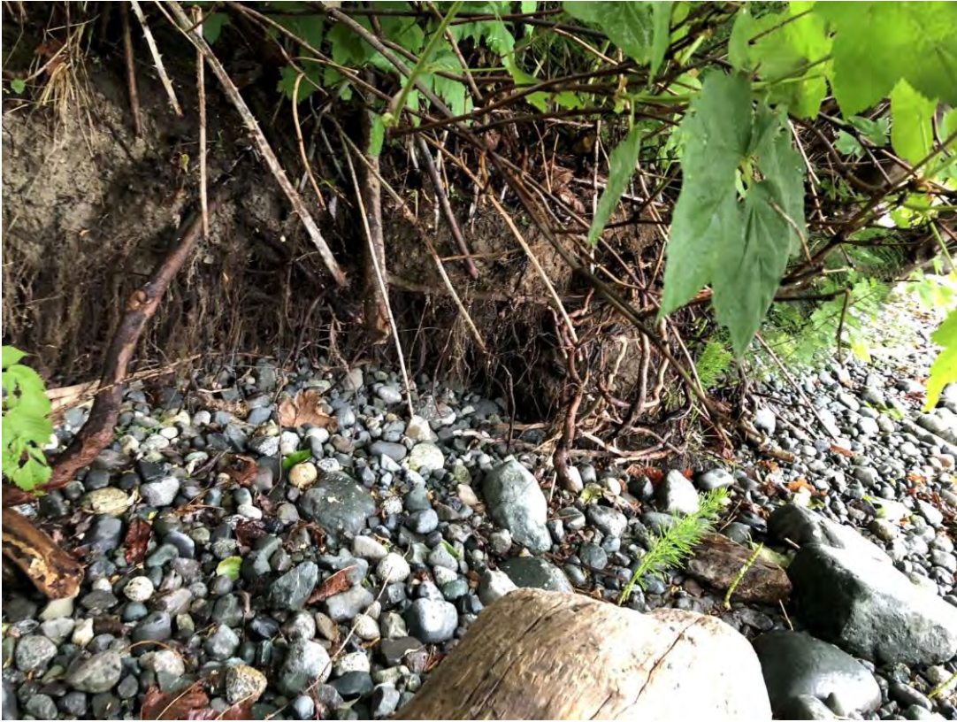
P07: Toe erosion near 4665 Discovery Dr.
