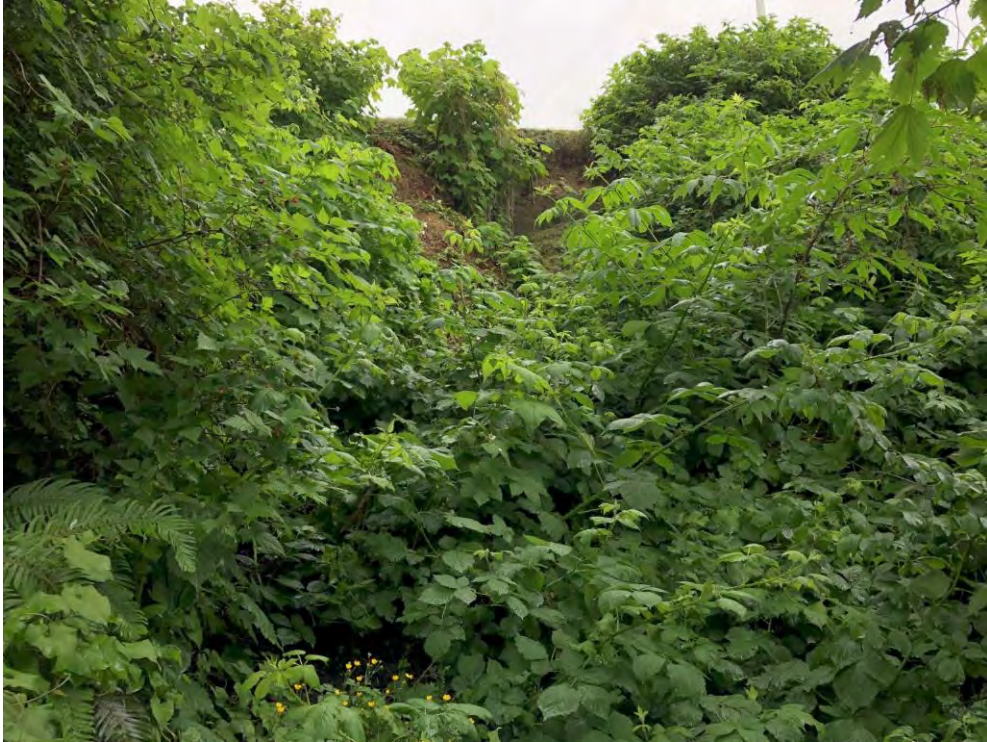
P44: Close up of crest erosion near 4365 Discovery Dr.
