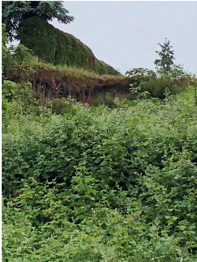
P04: Close up of crest erosion near 4685 Discovery Dr.
