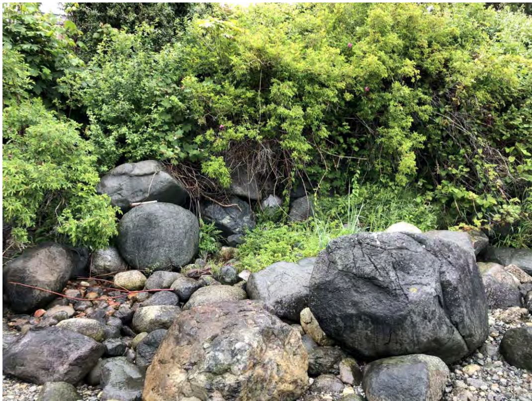
P55: Toe erosion near 4125 Discovery Dr.
