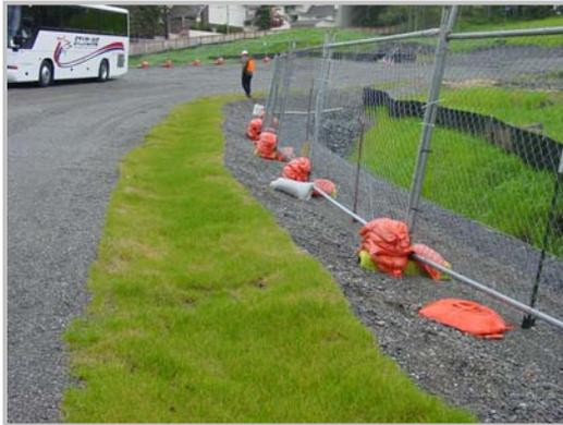
To address erosion and sediment control practices on construction sites, we recommend that the City prepare a detailed ESC brochure or pamphlet that would be distributed with every building permit application. The brochure would outline the City's expectations for ESC on construction sites as well as a discussion on the impacts to local watercourses and fish habitat if proper ESC practices are not followed. Source control practices such as minimizing cleared areas, timing
