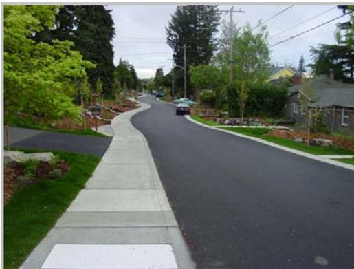
Rather than upgrading a road section to a typical urbanized section with curbs, gutters, catch basins and storm sewers, there may be an opportunity to implement alternative roadway design options for stormwater control, through the use of components such as porous pavements, vegetated swales, infiltration facilities and reduced impervious areas. These features have been used in other areas of the Pacific Northwest, most notably in Seattle, Washington as part of the Street Edge Alternative
