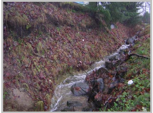
21. Ditch undergoing severe erosion
