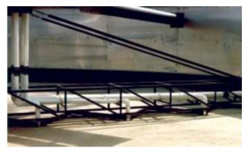
Individual sludge removal pipes for Type CR design.
