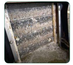
Wastewater passes through perforated panels while unwanted solids are removed.
