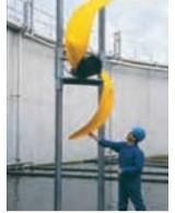
The most frequently-used installation method employed with the Flygt 4400 series mixers is the guide bar with the mixer being easily raised and lowered. This method gives easy accessibility for servicing.
