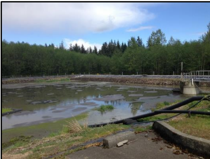
Photograph 2: A poly-lined storage lagoon at the City of Campbell River's Norm Wood Environmental Centre wastewater treatment plant. (April, 2015)
