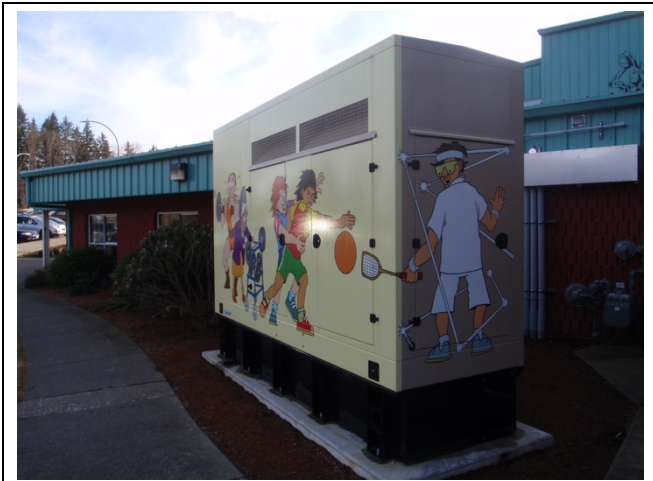
Photo 41 D5092.1 Emergency Generator
