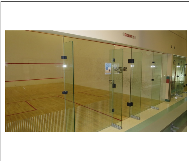
Photo 19 C1013 Non-Movable Court Glass Wall
