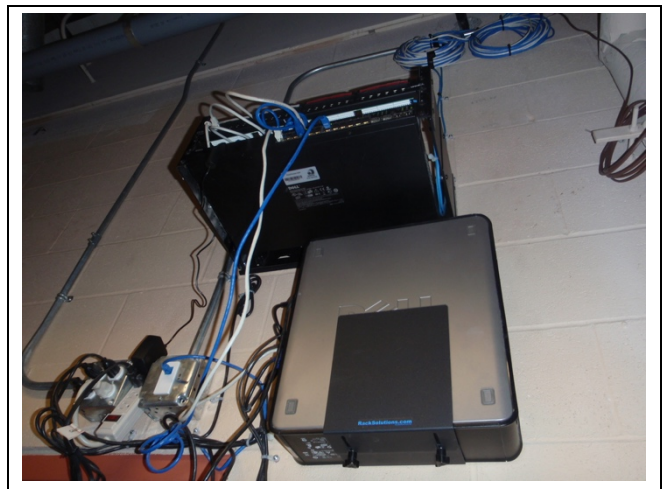
Photo 40 D5030 - Data & Telecom
