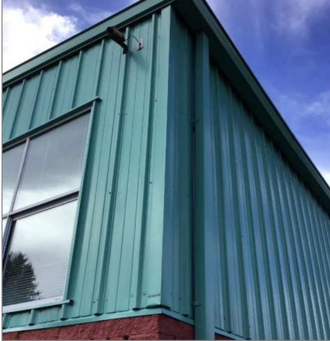
Figure 2.2 Wall Protection Wall cladding is exposed to rain fall.
