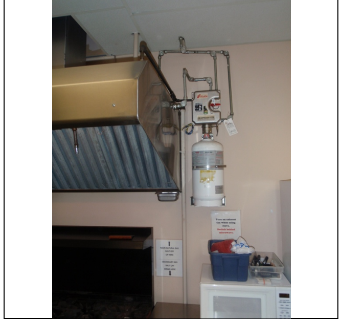
Photo 38 D4095 - Hood Fire Protection
