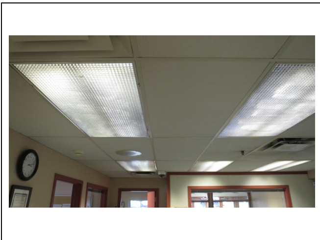
Photo 39 D5022.1 - Internal Lighting
