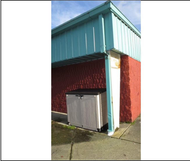
Photo 1 B1021 Steel I-beams require Painting
