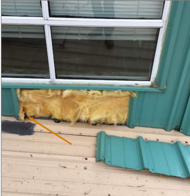
Figure 2.5 Cladding Insulation Bottom of insulation wet at pinch point of insulation blanket.
