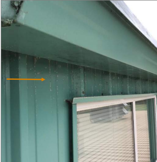
Figure 2.3 Cladding Corrosion Surface corrosion at protected cladding locations such as directly under gutters.
