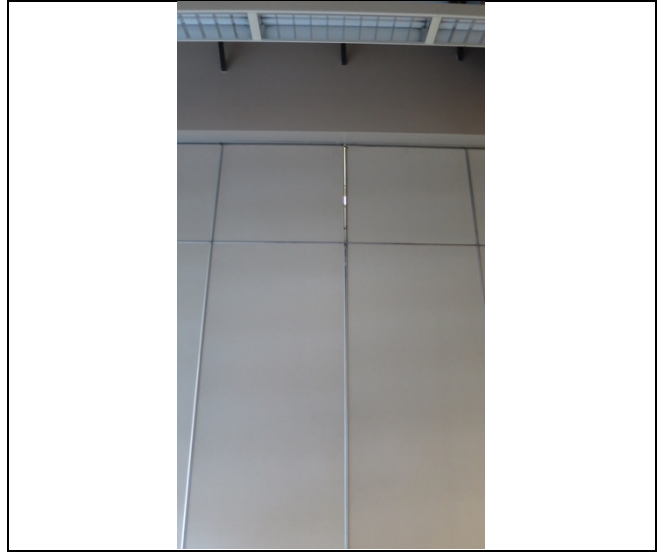
Photo 22 Activity Room Folding Partition-Requires maintenance
