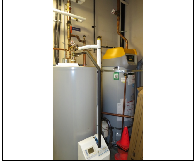
Photo 34 D2022 - Hot Water Service
