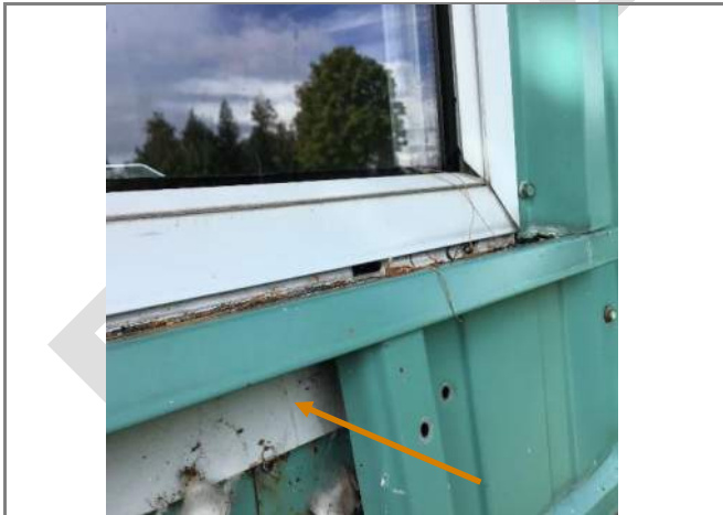
Figure 2.6 Window Sill Flashing Debris visible below the window sill flashing.
