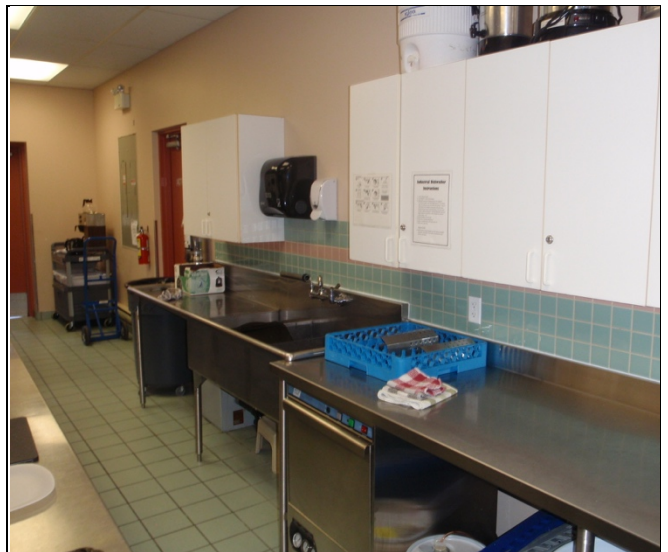
Photo 32 D2014 - Commercial Sinks
