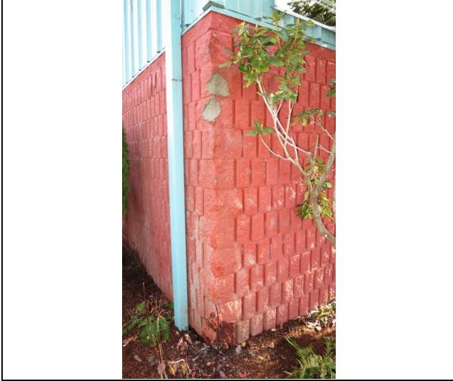
Photo 9 B2011 Water behind Masonry Block-Deteriorating Corner
