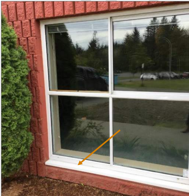
Figure 2.10 Window Sill Flashing
