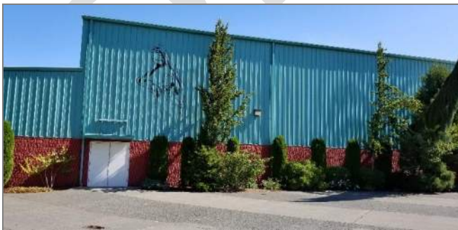
Figure 2.11 South West Elevation - Metal Cladding
