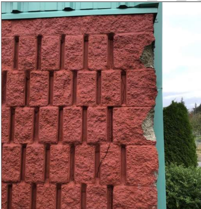
Figure 2.8 Block Wall Spalling at block wall corner and cracking noted.
