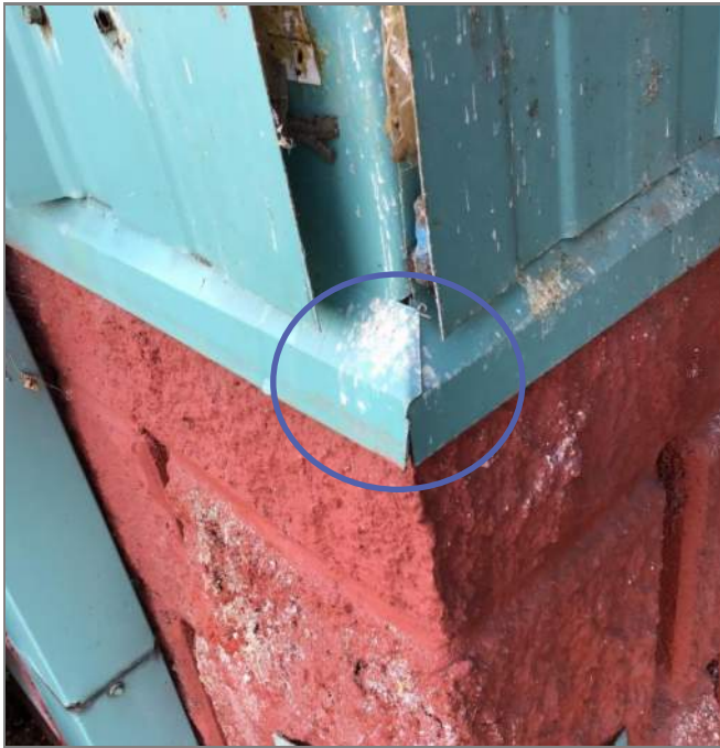
Figure 2.9 Cladding Sill Flashing
