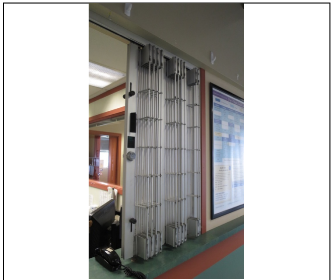
Photo 20 C1013 Lobby Security Grille
