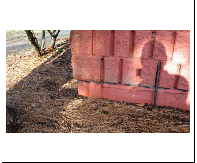
Photo 6 B2011 Water behind masonry Block
