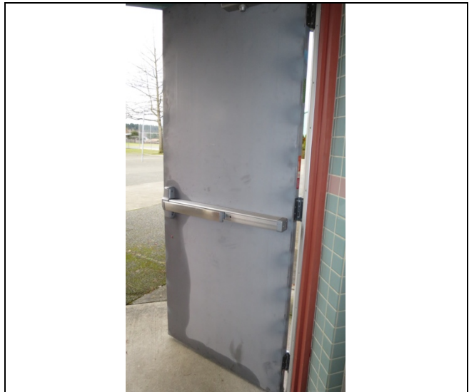
Photo 12 B2032 Exterior Doors require Paint
