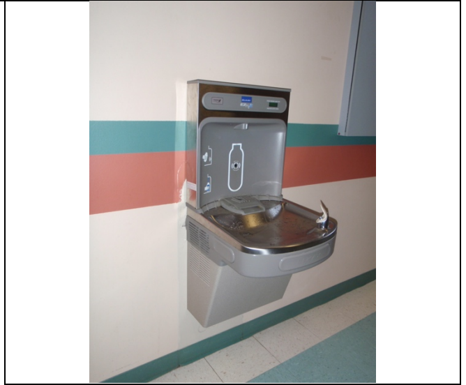
Photo 30 D2000 - Fountain & Water Bottle Station
