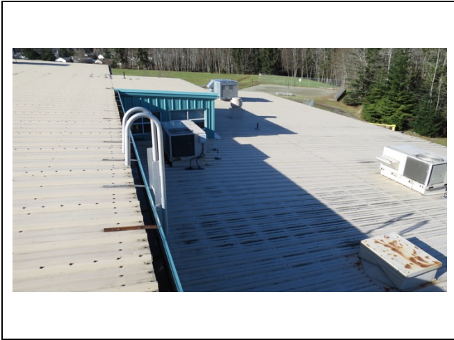
Photo 13 B3011 Metal Roofing
