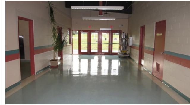
Photo 17 C1011 Painted Fixed Partitions
