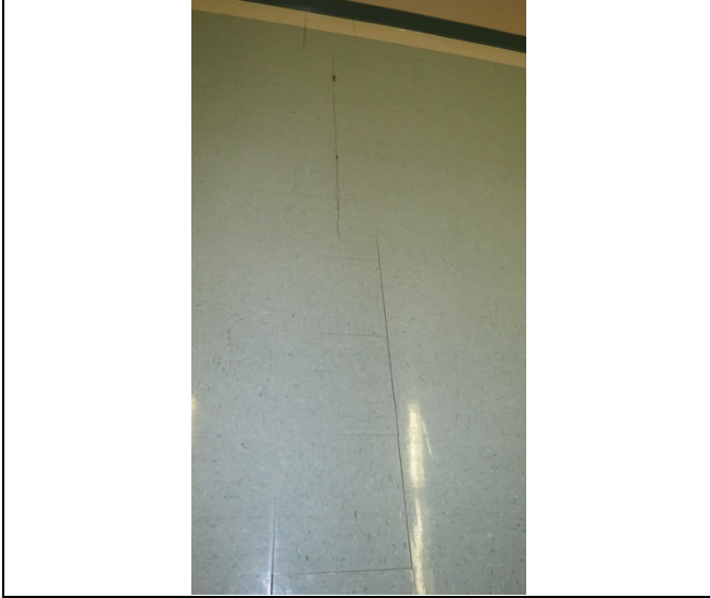
Photo 5 A1031 Crack in Slab-on-Grade near GL's 8 & D
