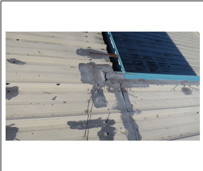
Photo 15 B3011 Metal Roof Repair
