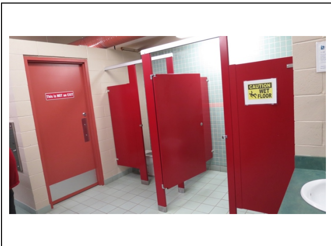
Photo 23 C1031 Toilet Partitions
