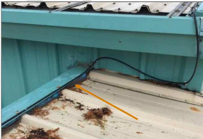
Figure 2.19 Roof Gaskets Deterioration of the foam roof edge gaskets.
