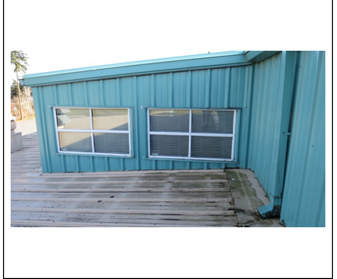
Photo 10 B2021 Exterior Windows
