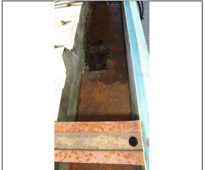
Photo 16 B3011 Rusting Gutter
