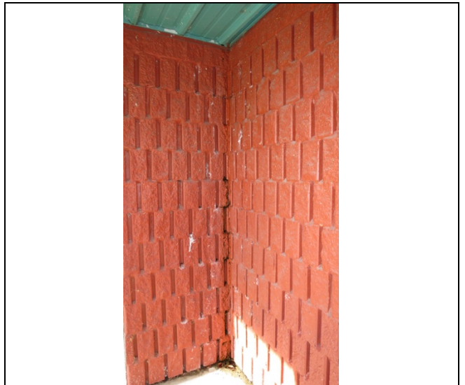
Photo 8 B2011 Roof Leak Water behind masonry Block
