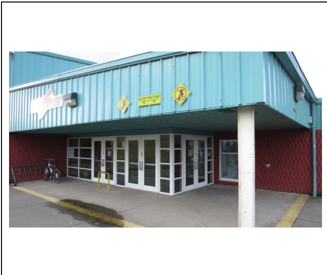
Photo 11 B2023 Storefront Assembly - Main Entry
