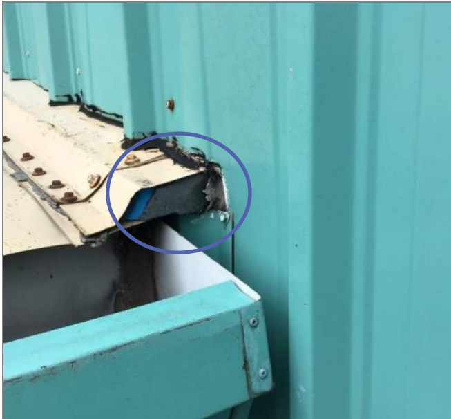
Figure 2.23 Roof Eave to Wall Junction
