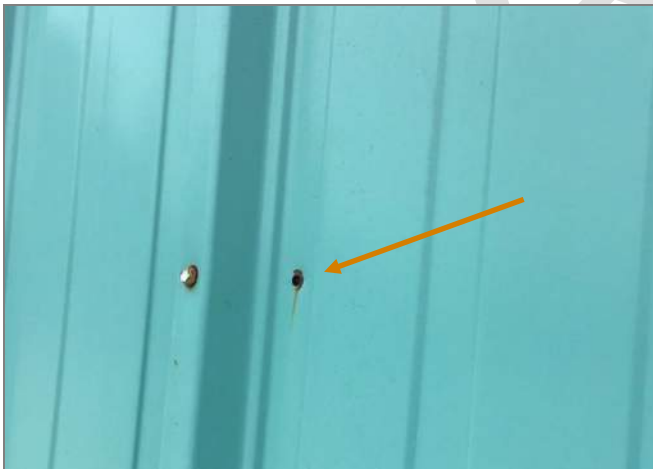
Figure 2.4 Cladding Fasteners Corrosion identified on fasteners and at fastener penetration.
