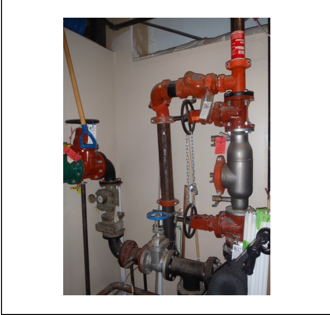
Photo 37 D4011 - Sprinkler Tree
