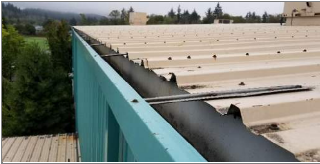
Figure 2.20 Roof Fasteners Surface corrosion on exposed metal fasteners.
