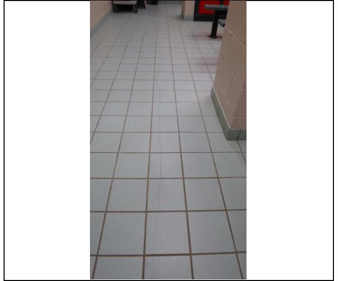
Photo 2 A1031 Crack in Slab-on-Grade near GL's 9.1 & Q
