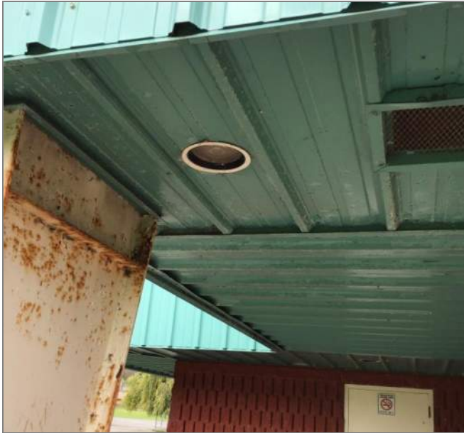
Figure 2.7 Soffits Corrosion of the metal soffits.
