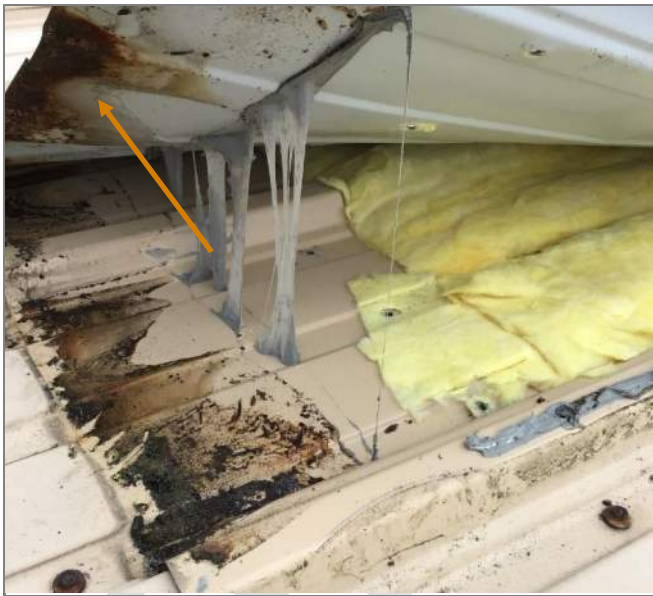
Figure 2.21 Roof Corrosion Corrosion of the metal roof panel.
