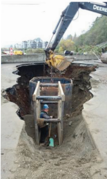
Crews work at the Anchor Inn to complete connections for the new pump station.
