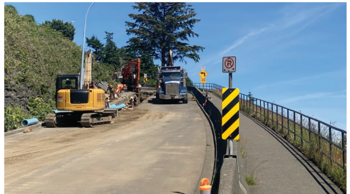
Crews work at the top of Rockland Road hill to install a new water forcemain – a key first piece of the project work.
