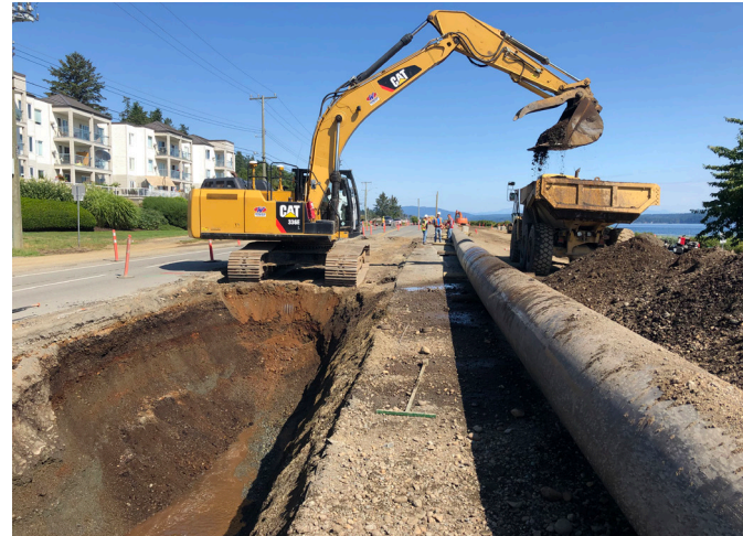
Forcemain installation has started along Hwy 19a near Rockland Rd.
