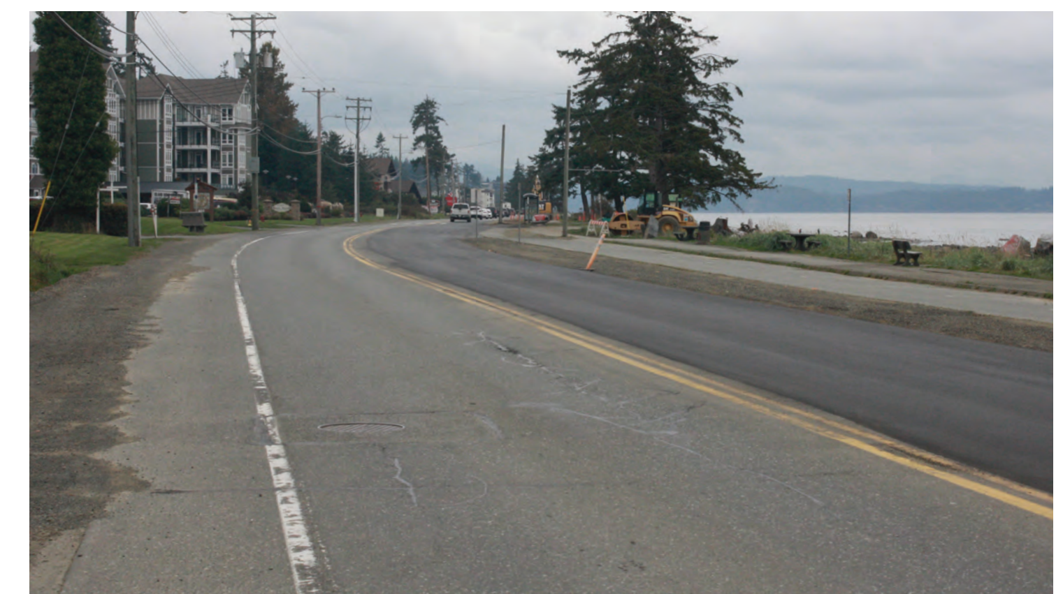
Photos from 2019 construction
