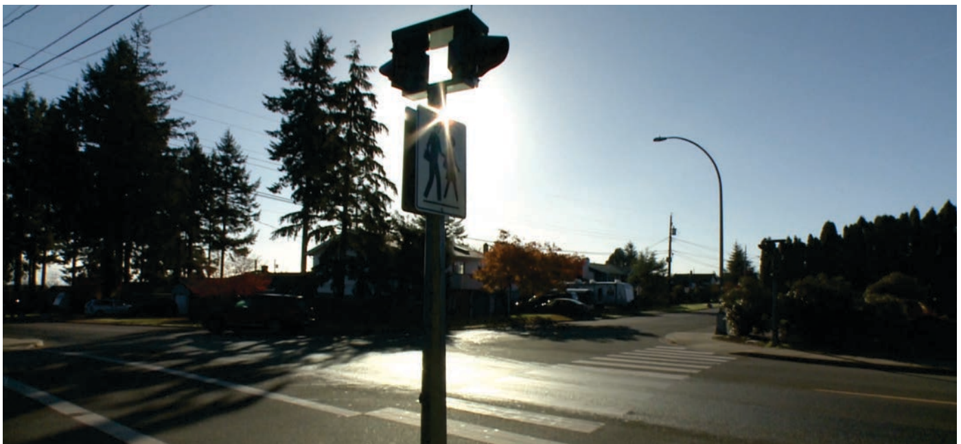
Solar-powered flashing pedestrian traffic signals
