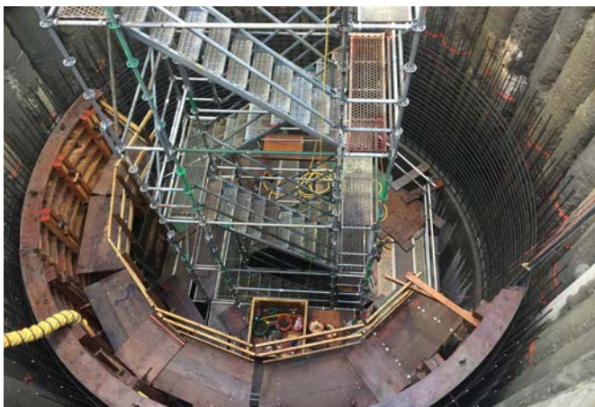
Campbell River Water Supply Project - Phase 2
