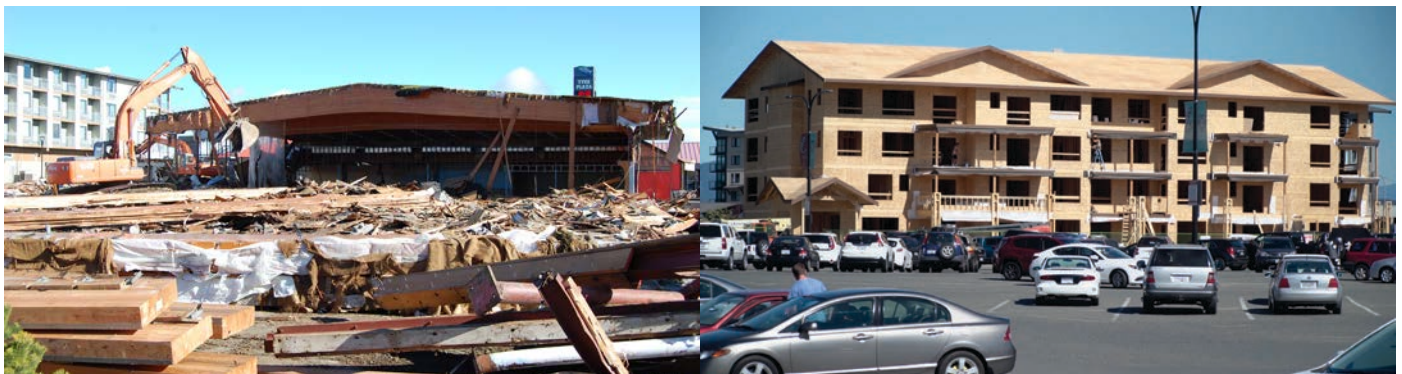
Before and after: demolition and construction in Tye Plaza
