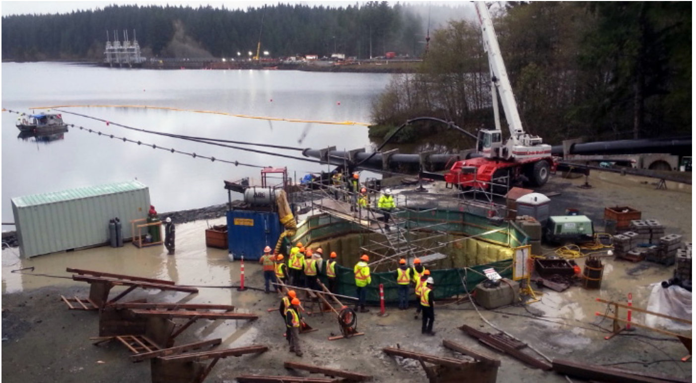
Campbell River Water Supply Project - Phase 2
