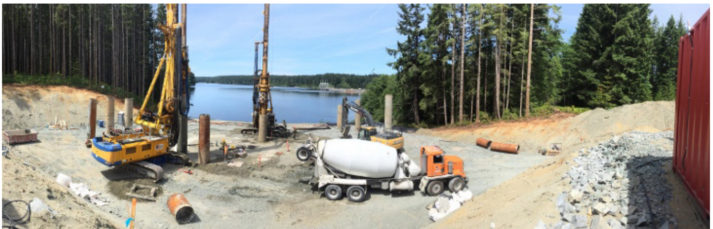
Campbell River Water Supply Project - Phase 2
