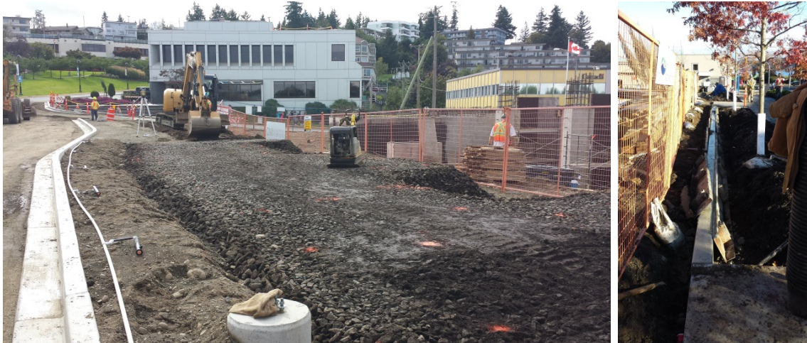
Figure 12. The public street component of the Seymour Pacific development on St. Ann’s Street included the installation of structural soils beneath the sidewalk to increase the volume of soil available for the Scarlet Oaks planted in the roadside.
