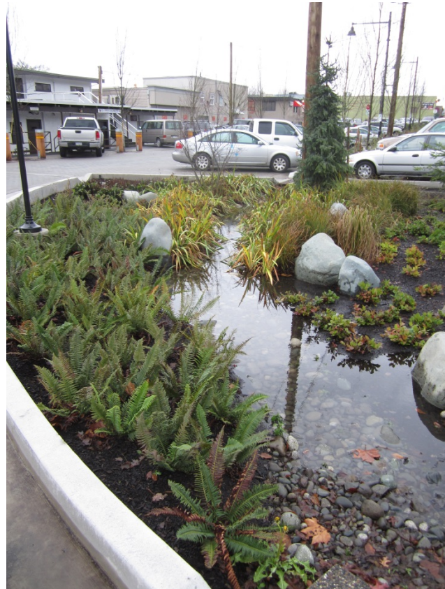
Figure 13. Raingarden capturing stormwater and allowing infiltration into the soil.
