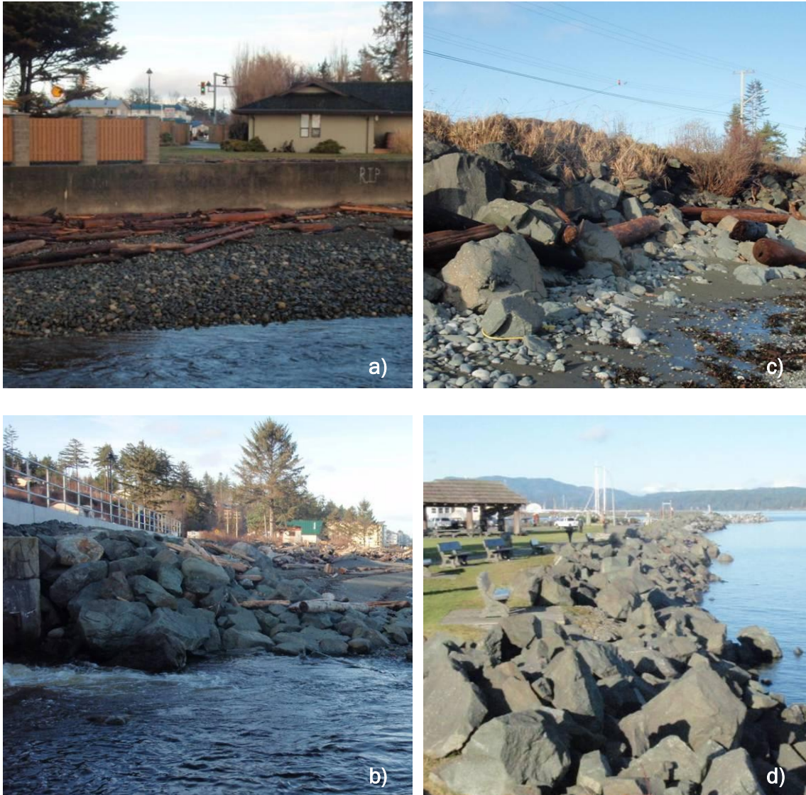
Figure 9. Typical bank armoring along the CoCR foreshore; a) vertical concrete wall at Willow Creek, b) loc-bloc and rock wall protection along new Island Highway South at Simms Creek, c) steep failing riprap near the end of Dahl Road, and d) rock riprap lined shoreline at Frank James Park (all photos 17 January 2011).
