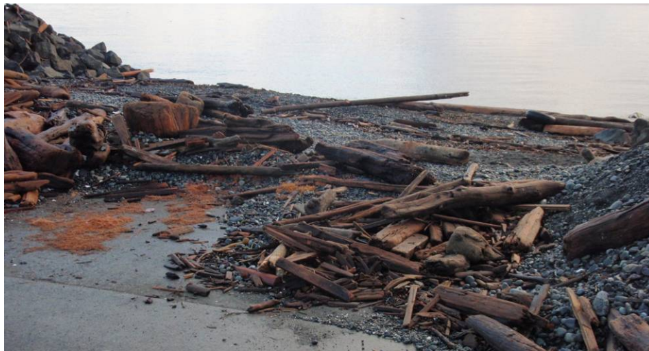
Photo B-3. Sediment and debris clogging Ken Forde boat ramp on 17 January 2011. The ramp was cleared in late-December, 2011.
