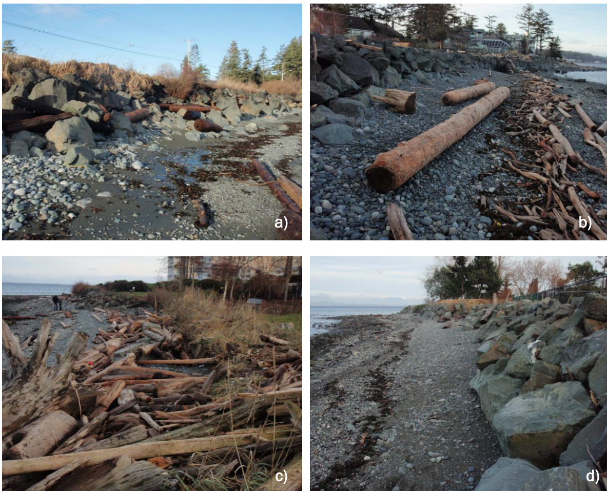
Figure 13. Photos showing conditions at the lower priority sites (see Table 17): a) along shore near Twillingate Road, b) Larwood Park, c) Adams Park, and d) Frank James Park (photos taken 17 January, 2011).
