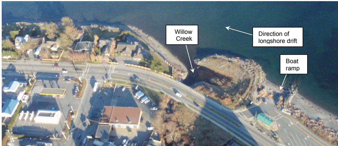
Photo B-4. Oblique aerial view of Ken Forde Boat Ramp (photo taken 18 January 2011).
