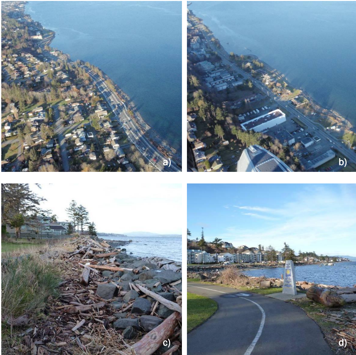
Figure A-6. Various photos showing shoreline conditions from McCallum Park to Rotary Park (photos taken 17 January 2011).
