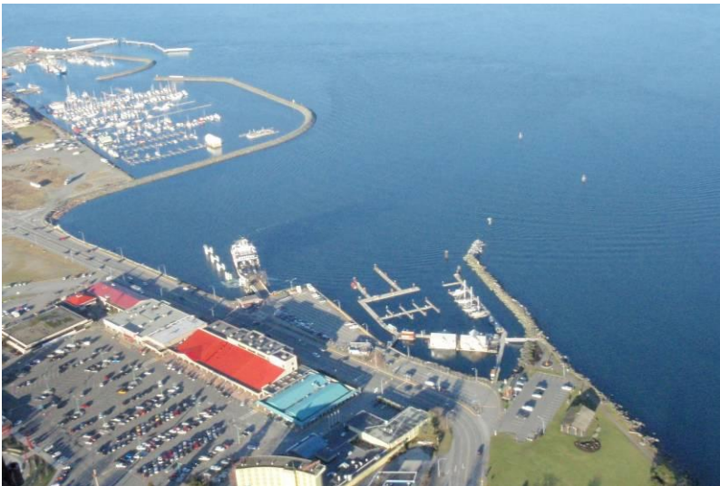
Photo 2. Oblique aerial photo of the breakwaters and jetties installed at the BC Ferries terminal and the Discovery Harbour Marina (photo 18 January 2010).
