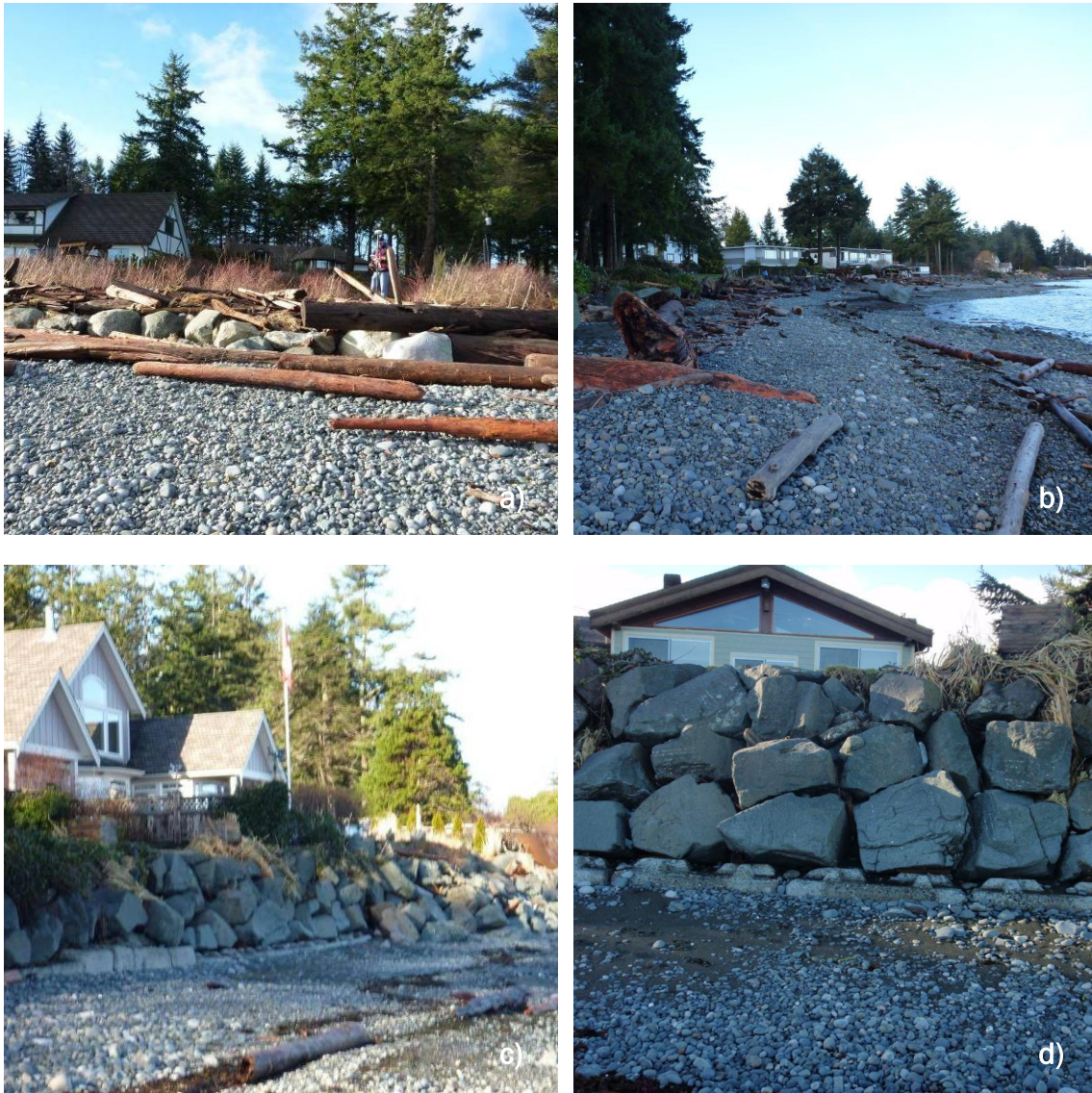
Figure A-4. Various photos showing shoreline conditions north of Ocean Grove Road (photos taken 17 January 2011).
