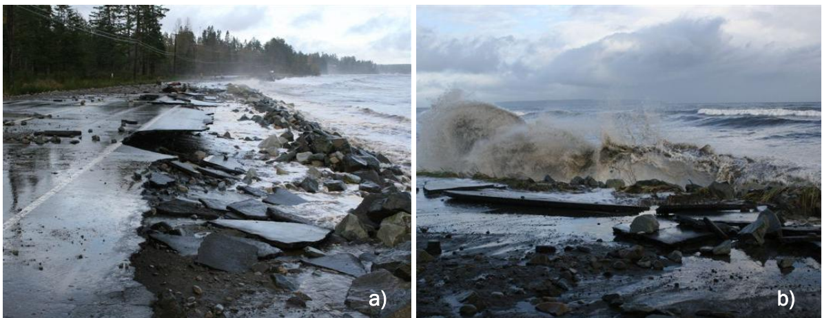
Figure A-20. Photos showing damage to Highway 19A during 2007 storm.
