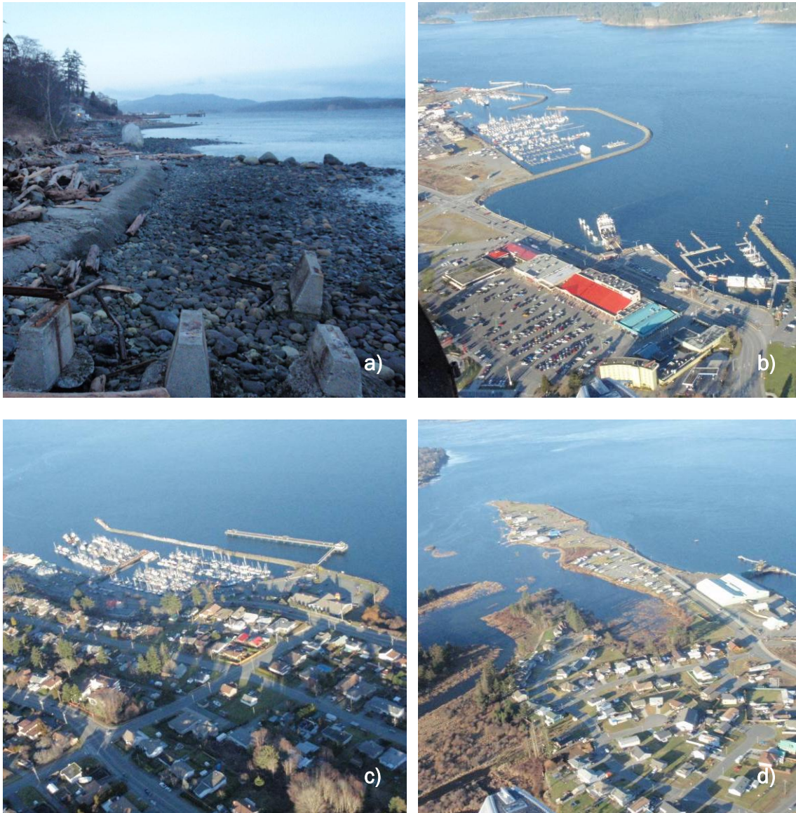
Figure A-8. Various photos showing shoreline conditions from Hidden Harbour Park to Tye Spit (photos taken 17 January 2011).
