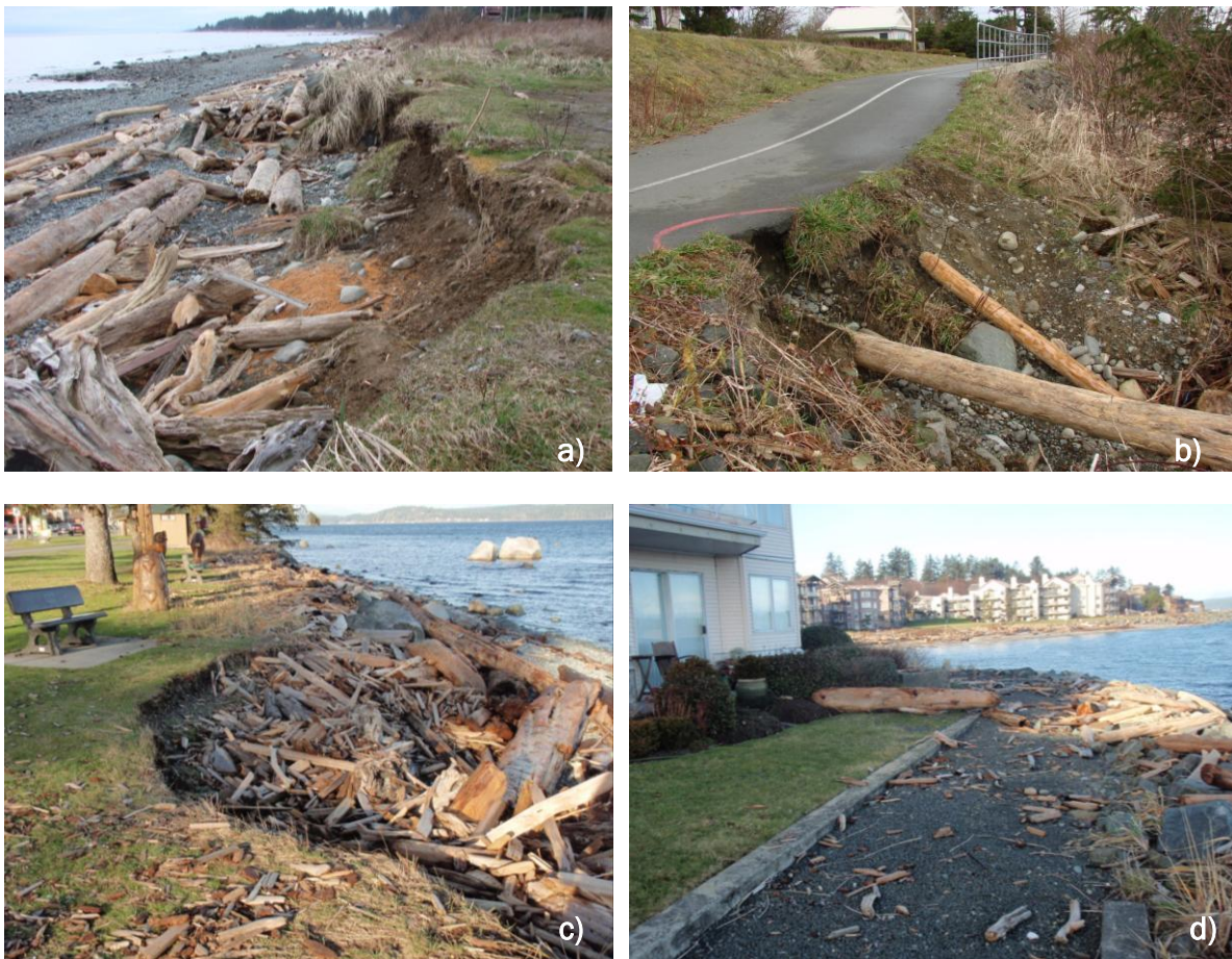
Figure 12. Photos showing conditions at the high priority sites (see Table 16): a) south of Maryland Road, b) south of Twillingate Road, c) Rotary Beach Park, and d) Seaside Estates (photos 17 January, 2011).
