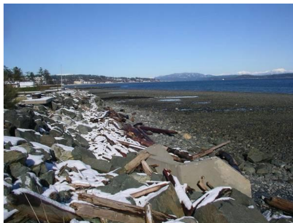
Photo 7. Typical shoreline armoring in the Willow Point Reach.
