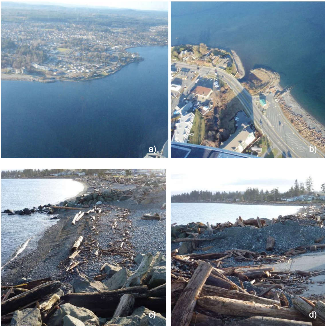
Figure A-5. Various photos showing shoreline conditions in the Willow Point area (a and b) and Ken Forde Boat Launch (c and d) (photos taken 17 January 2011).
