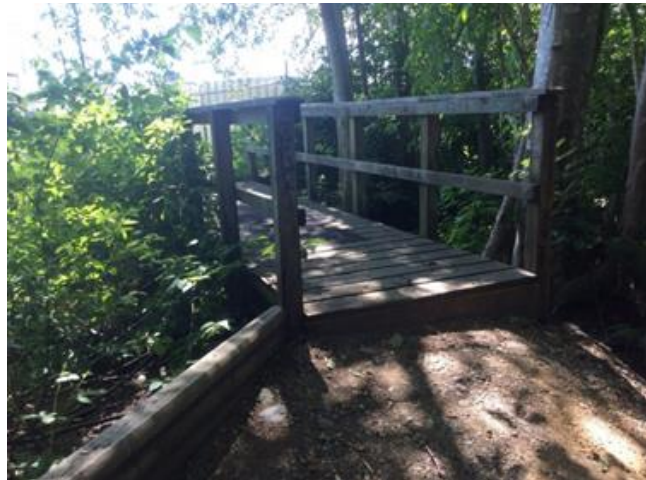
i). Bridge in good repair, top view, B05, on May 24, 2016.
