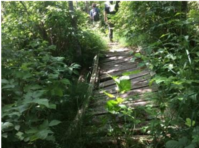
m). Bridge in poor repair, top view, B09, on May 24, 2016.
