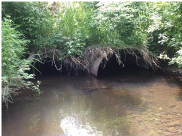
c). Culvert from Homewood, C02, on May 24, 2016.
