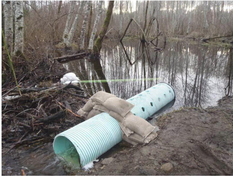
Figure 3. Completed installation of a drainage pipe in the beaver dam in EU2a, 2010 (Martin, pers. comm. 2016).
