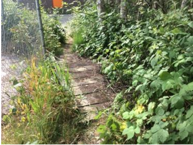
k). Bridge in moderate repair, top view, B07, on May 26, 2016.
