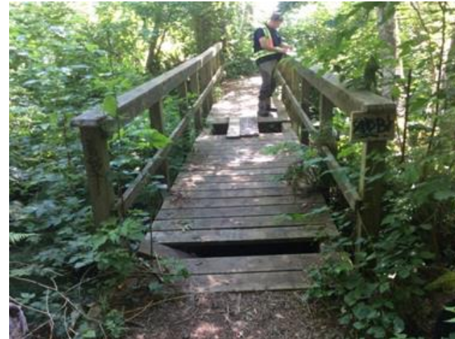
d). Bridge in poor repair, top view, B02, on May 24, 2016.
