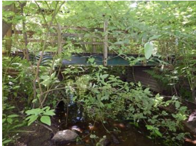
c). Bridge in poor repair, side view, B02, on May 24, 2016.
