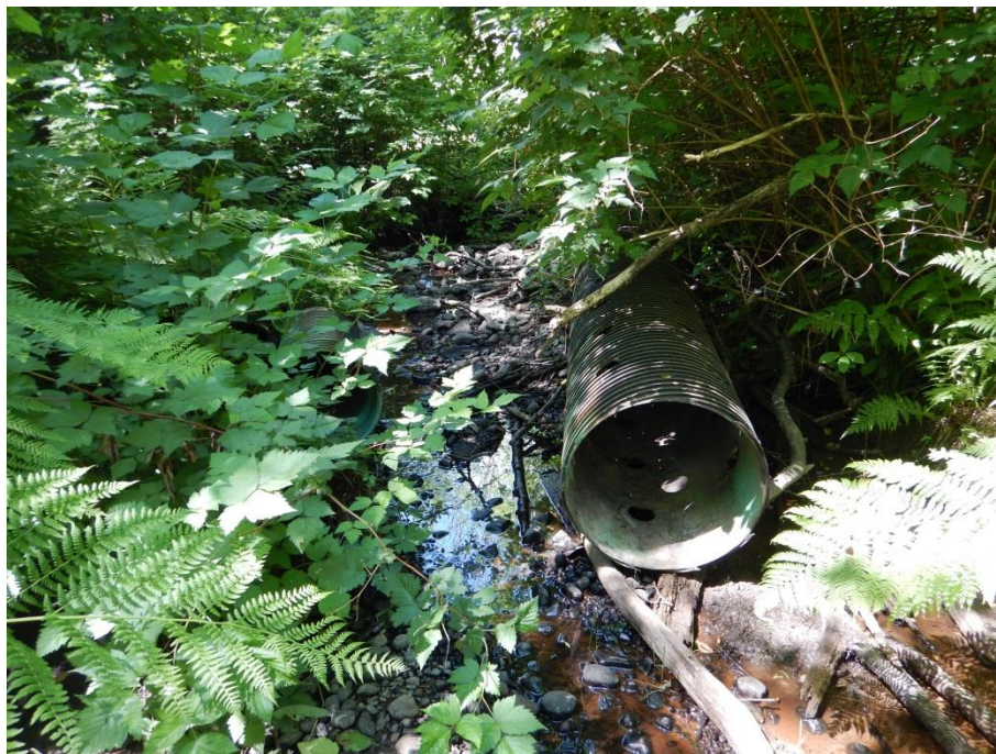
Figure 4. Drainage pipe washed downstream of beaver dam in EU2a, May 24, 2016.
