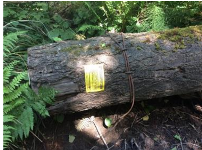
d). Anchored LWD on May 24, 2016.
