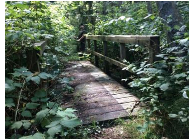
n). Bridge in moderate repair, good condition but grown over and requires new tread, top view, B11, on July 14, 2016.
