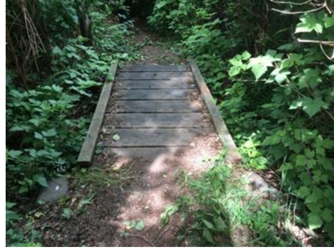
l). Bridge in moderate repair, top view, B08, on May 26, 2016.
