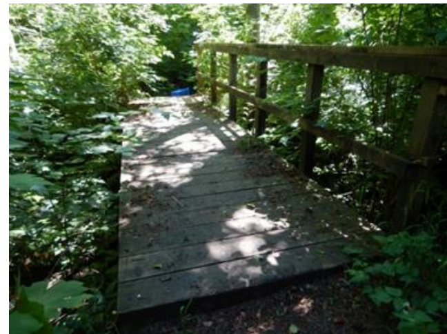
j). Bridge in moderate repair, top view, B06, on May 24, 2016.
