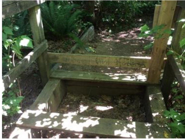
g). Bridge in poor repair, graffiti, top view, B04, on May 24, 2016.
