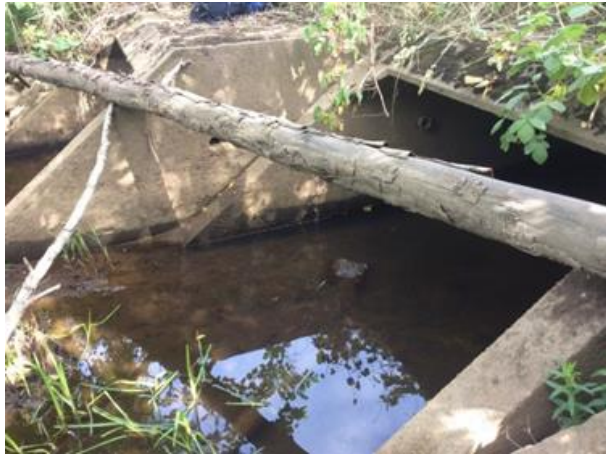
a). 16th double box culvert, C01, on May 24, 2016.
