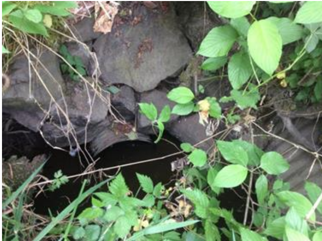
e). Storm drain from Homewood, SD02, on May 26, 2016.
