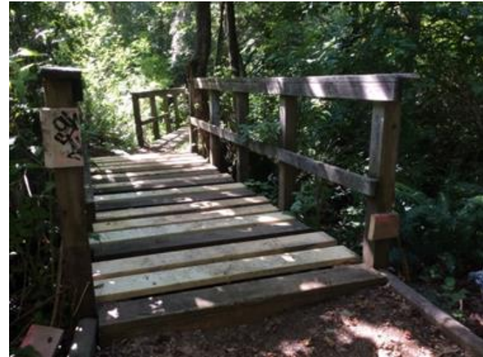
h). Bridge repairs, top view, B04, on July 14, 2016.
