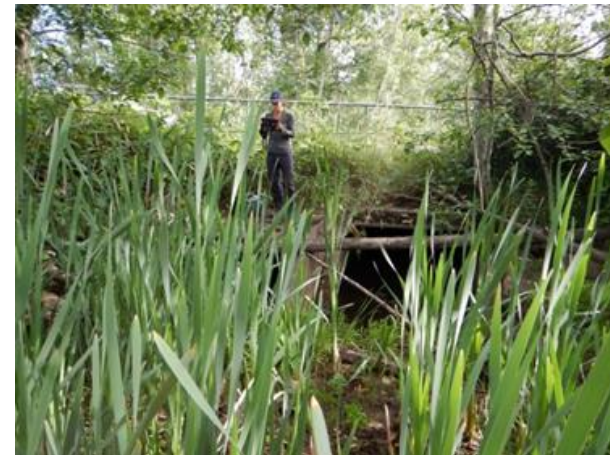
b). 16th double box culvert, C01, on May 24, 2016.
