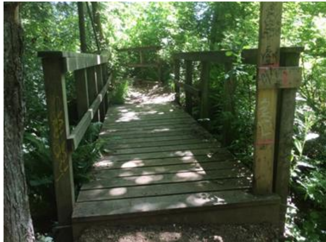
e). Bridge in moderate repair, top view, B03, on May 24, 2016.
