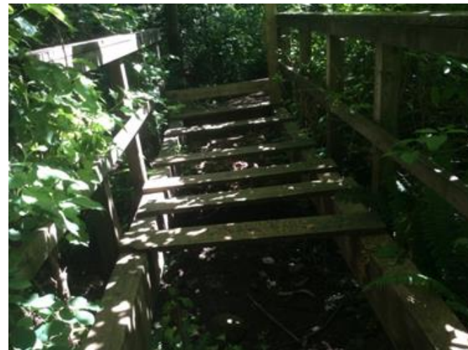
f). Bridge in poor repair, top view, B04, on May 24, 2016.
