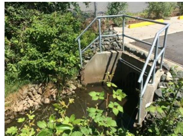
d). Storm drain from 12th, SD01, on May 24, 2016.
