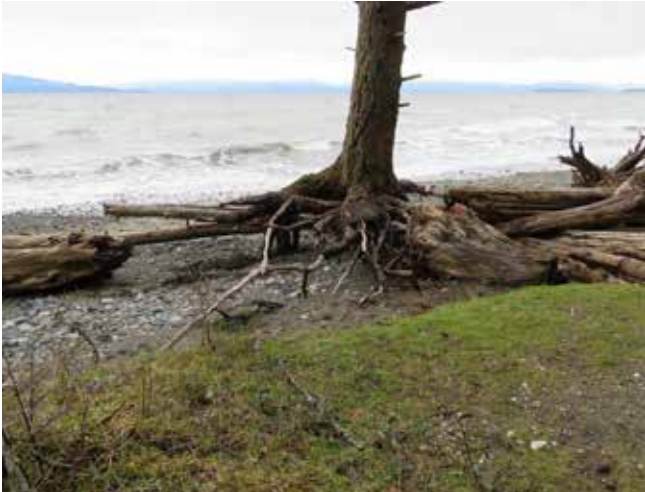
Shoreline erosion. Parksville, BC (Credit: Sanctuary Studios)
