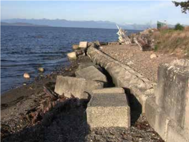
Seawall erosion failure. Parksville, BC (Credit: Sanctuary Studios)
