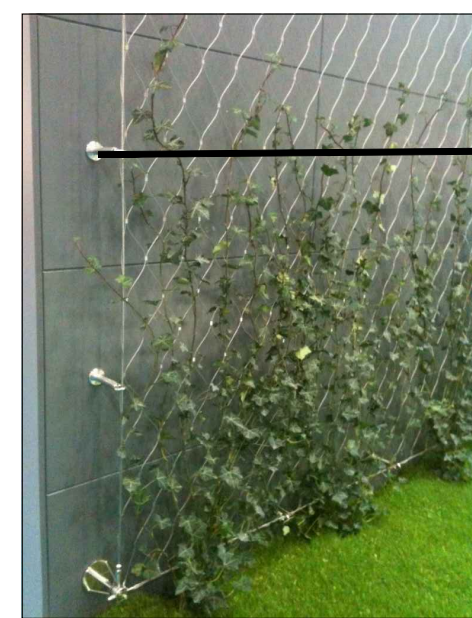
PROPOSED ATTACHED SYSTEM FOR WIRE TRELLIS
