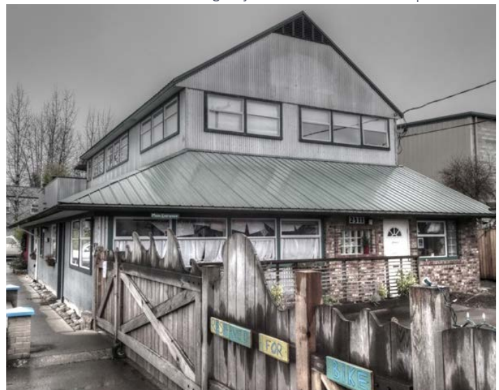
Tin Town, Courtenay: the consistent metal-clad design theme of this complex of live/work units creates a memorable industrially-themed architecture.
