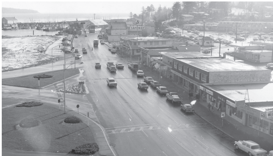
Lower Shoppers Row in yesteryear. The wide expanse of highway is stark when compared to today's street with wide sidewalks, curb bulge-outs, street trees and pedestrian crossings.
