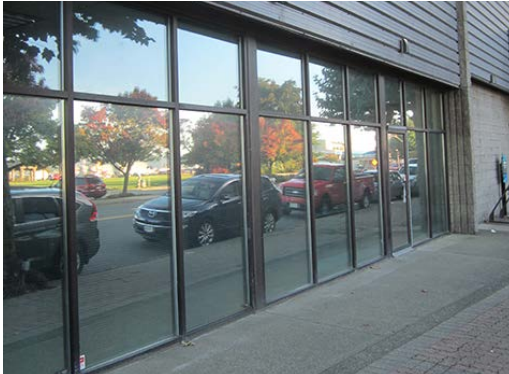
Lack of colour, architectural detail and obscure glazing present a unwelcoming and cold frontage to pedestrians. Private offices at ground floor level are not a good use for a building in a principal shopping street.
