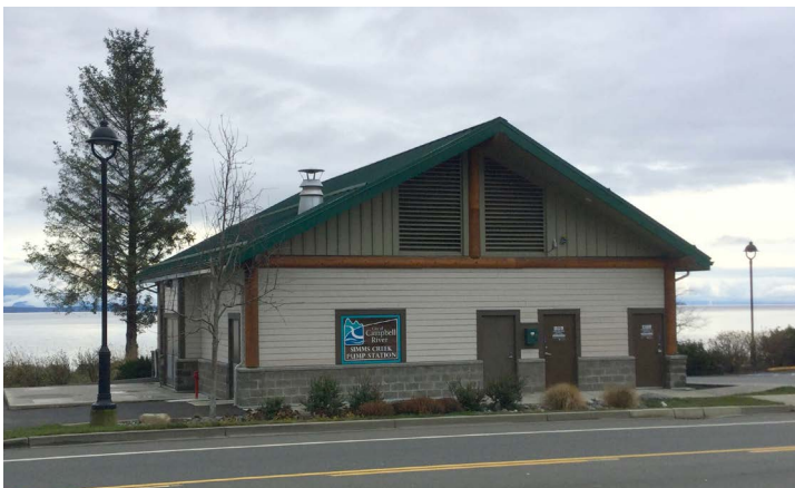
Simms Creek Pump Station
