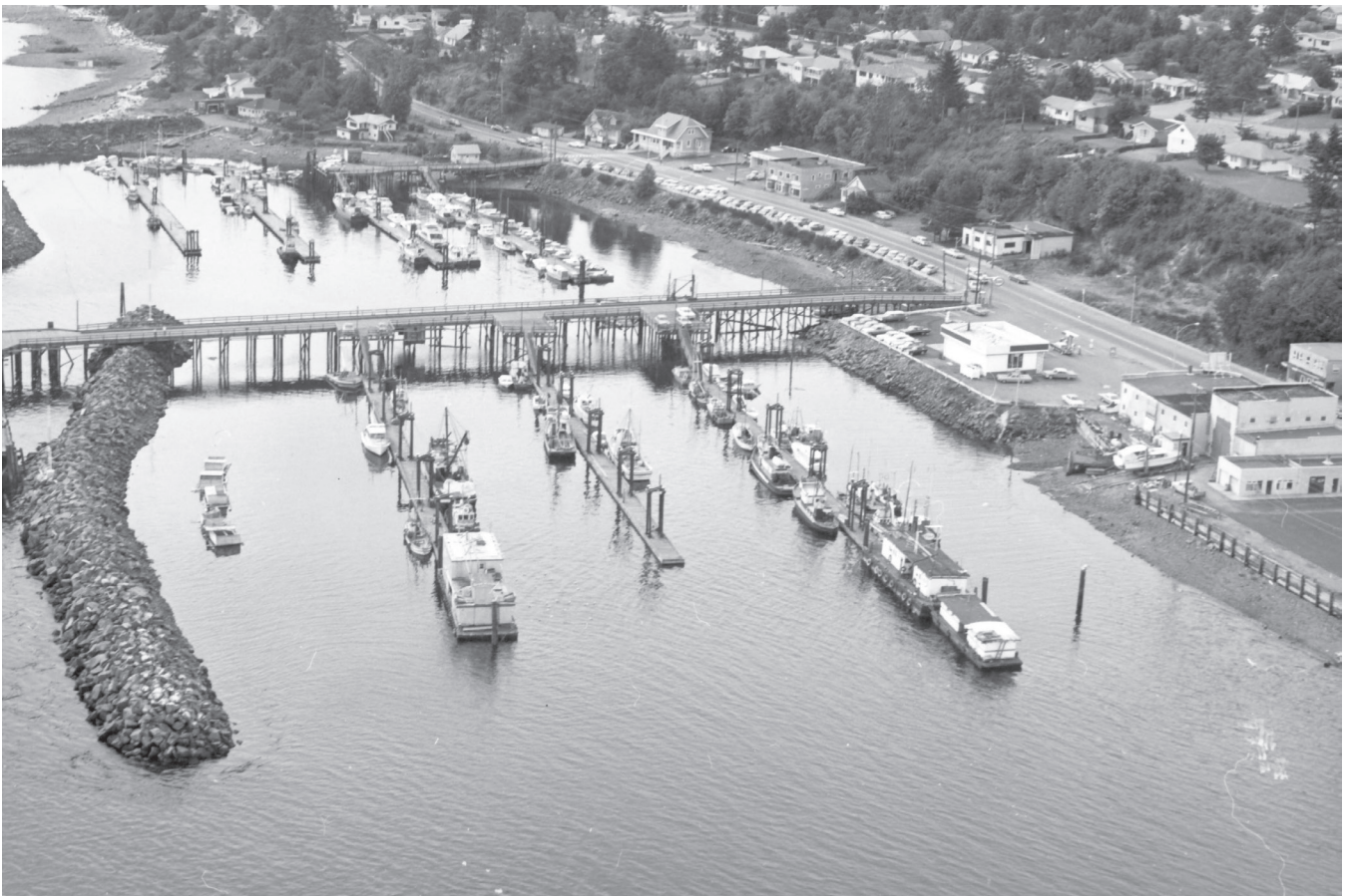
Historic image showing Pier Street. The boat slipway over which the waterfront walkway passes (“Shipyard Bridge”) is visible lower right in its operational condition.
