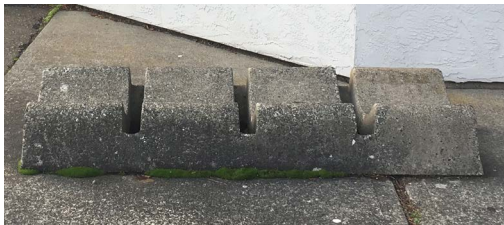
This bike parking block is an unattractive monolith and a possible trip hazard.
