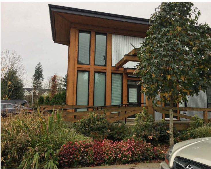
Heavy timber and corrugated metal combine to create an attractive modern building with a stylish industrial reference. Fort Langley, BC.
