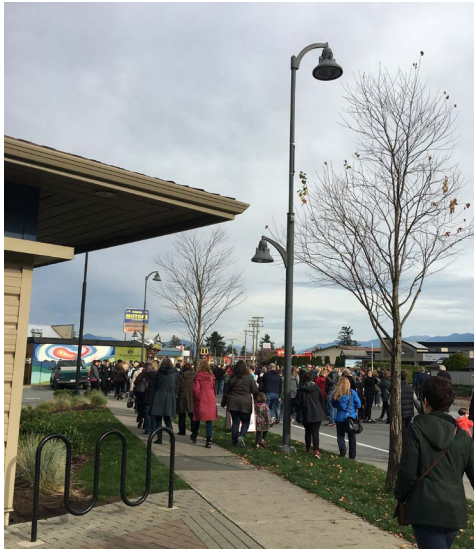
Two-level street lighting.
