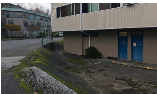
This transition between two elevations was poorly implemented and is now both unsafe and unsightly for pedestrians.
