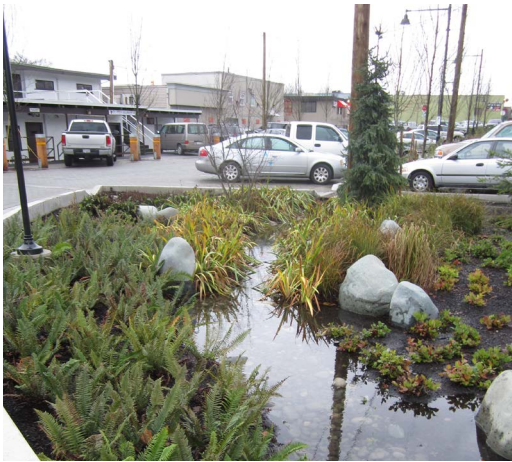
This beautiful raingarden uses native west coast plants, but also serves a valuable infrastructure purpose, slowing the discharge of rainwater into the storm drains.
