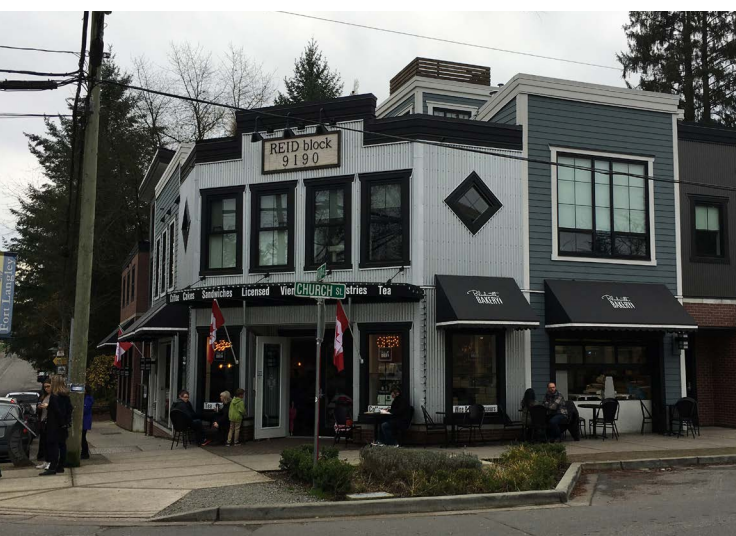
While clean and functionally modern, this historic building's appearance has been well preserved. Fort Langley, BC.
