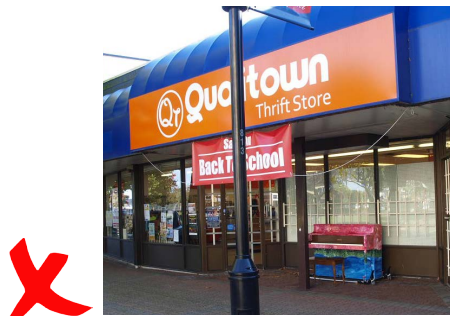
This fascia sign on the front of an awning is large and obtrusive, compounded by the inappropriate banner hanging beneath.
