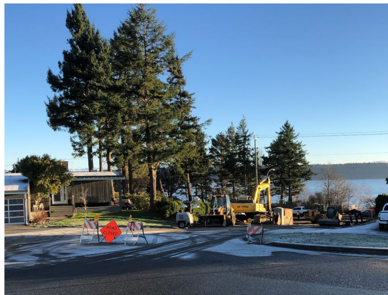
Construction at the 1st Ave. intersection
