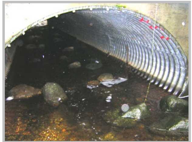
14. Jubilee Way east of Holmathco Drive CSP arch culvert
