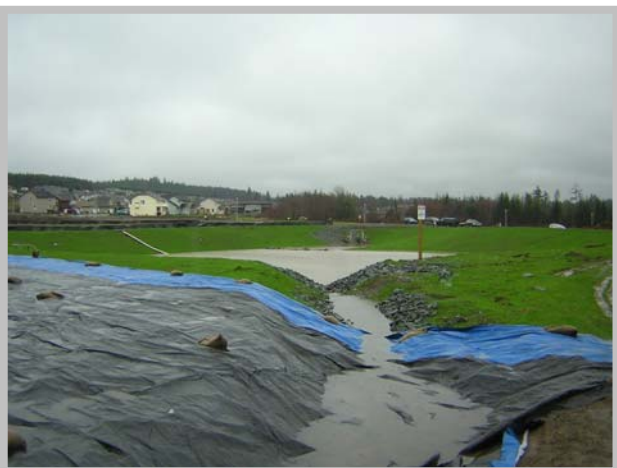
15. New detention pond under construction
