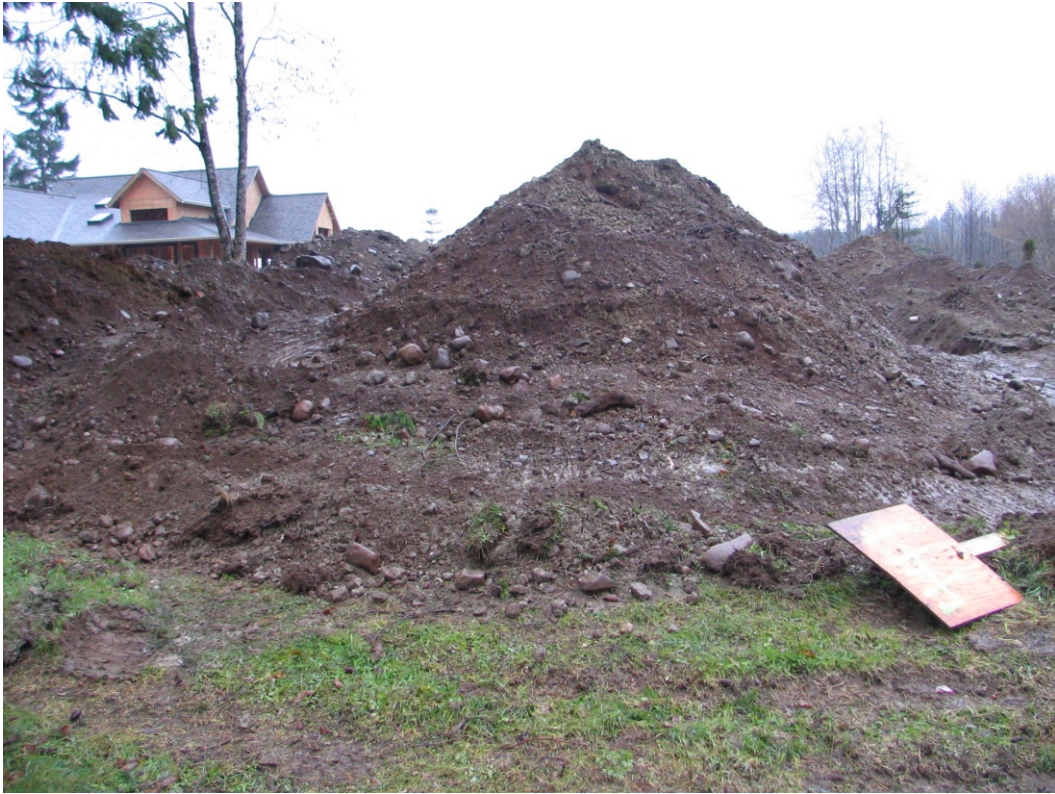
Photo 1. Excavated gravelly loamy sand unit (Dashwood soil) on Twillingate Road, south of Willow Creek. (December 7th, 2004)
