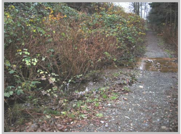
19. Springbok Road pond discharge over path
