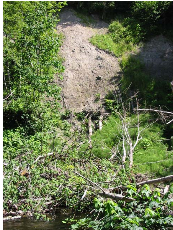
Photo 6: A thick section of silty sediments exposed at the west end of the study area.
