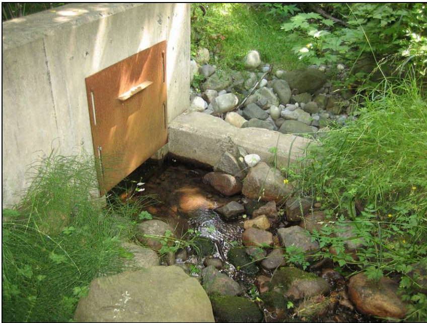
Diversion (bifurcation) structure on Haig Brown's Kingfisher Creek; low flows pass through the orifice on the left and high flows pass over the concrete weir to the rock-lined channel to the right
