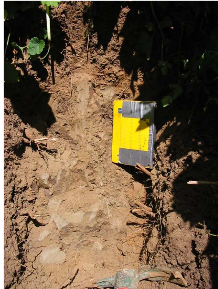
Photo 4: Fairbridge Soil exposed in a roadcut along Nursery Road consists of dense silt. Yellow notebook is 0.2m tall.
