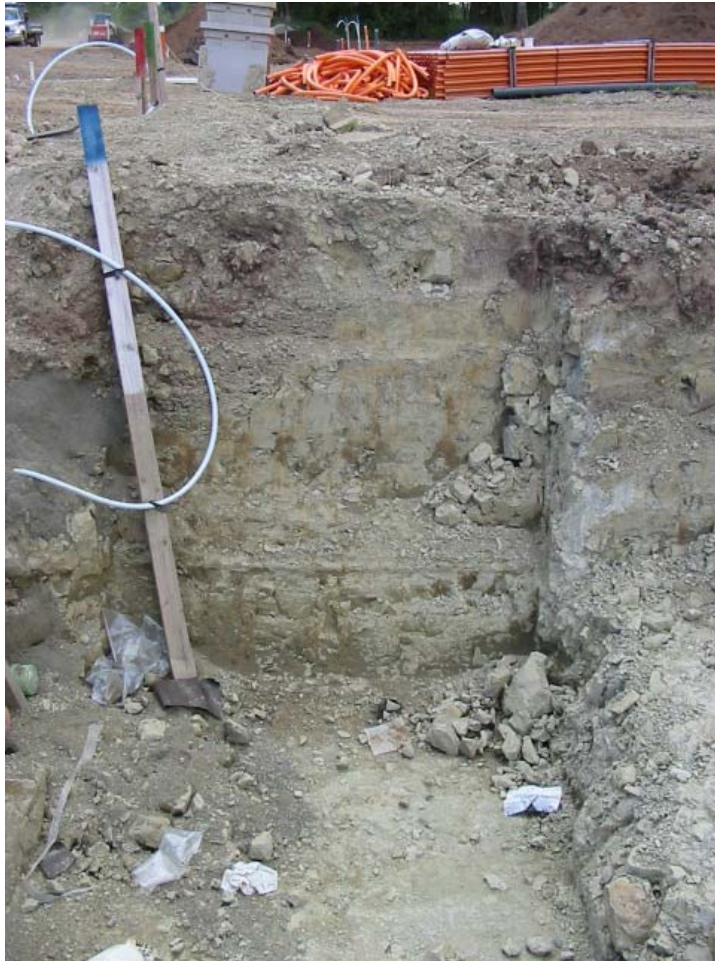
Photo 7: Fairbridge soil consisting of dense silt and clay exposed at a new residential development west of Cheviot Road.
