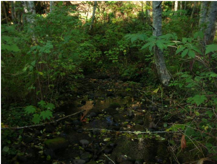
Photo 12. Downstream view of habitat downstream of the perched culvert in Haig Brown Kingfisher Creek where construction of rock riffles would assist passage over a wider range of stream flows (Oct 16 06).
