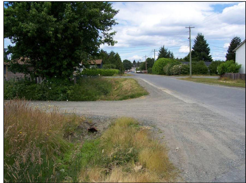
Typical Campbellton residential area, along 17 th Avenue; note use of ditches and culverts
