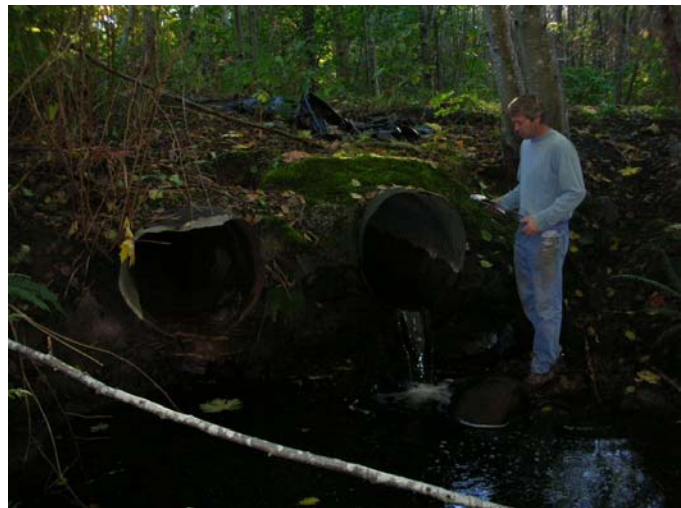
Photo 11. Upstream view of perched culvert at the forestry road crossing approximately 650 m upstream of the east/west fork junction (Oct 06).
