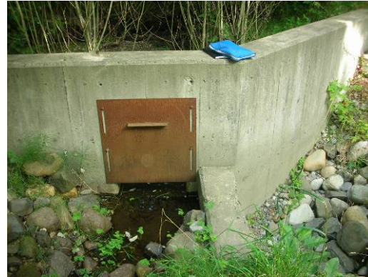
Photo 6. Downstream view of the bifurcation structure in HBKC East upstream of 14th Ave. Low flows proceed to top of picture and overflow to the right of the photo (August 06).
