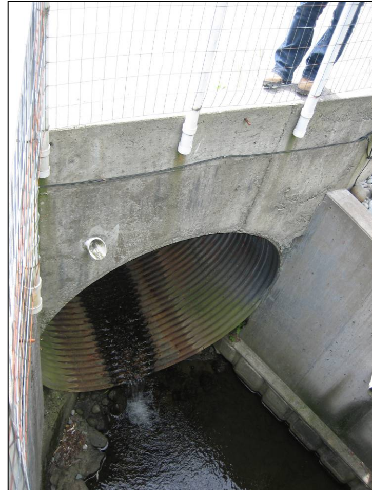
Outfall CR7; 2000mm diameter CMP
