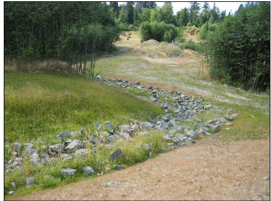
Riprap-lined channel servicing new Sequoia Springs development in upper Haig Brown's Kingfisher Creek watershed
