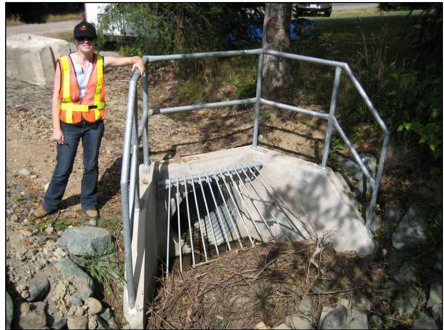
New headwall with trash rack on west end of Treelane Road
