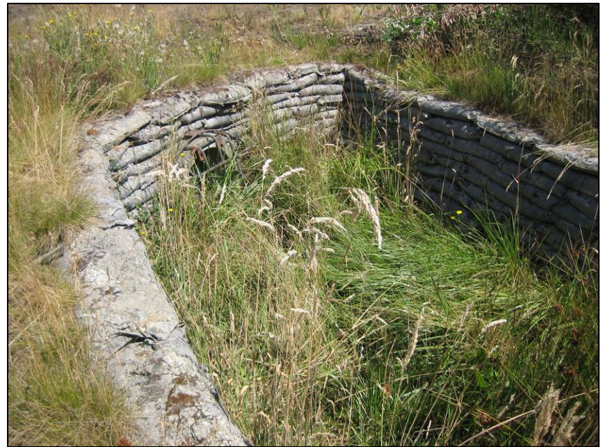
Outlet structure for water quality pond along Highway 19, near 14 th and Willow
