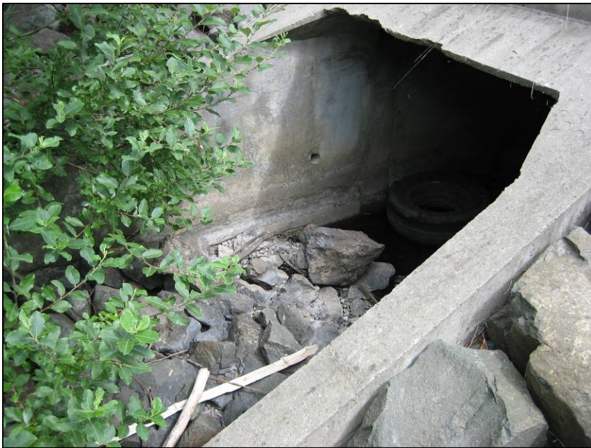
Box culvert under Campbell River Road; Haig Brown's Kingfisher Creek
