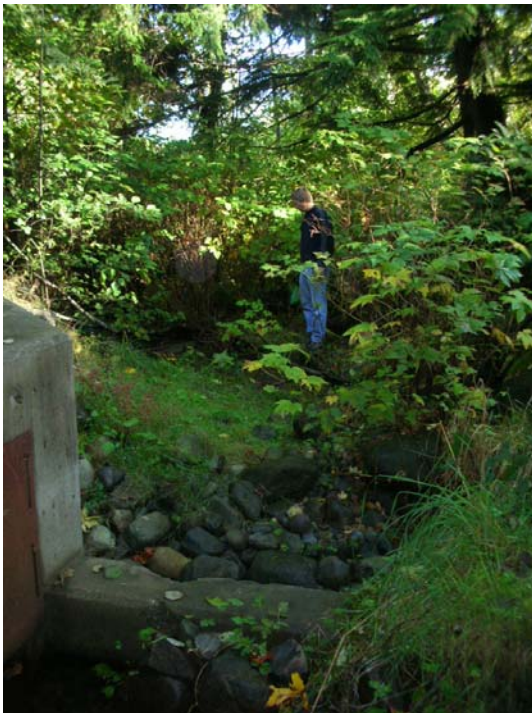
Photo 13. Downstream view of the high flow channel immediately downstream of the bifurcation structure illustrating cobble/boulder lined plunge pool and grassy overland undefined channel section downstream that has potential to strand migrating salmonids (Oct 06).
