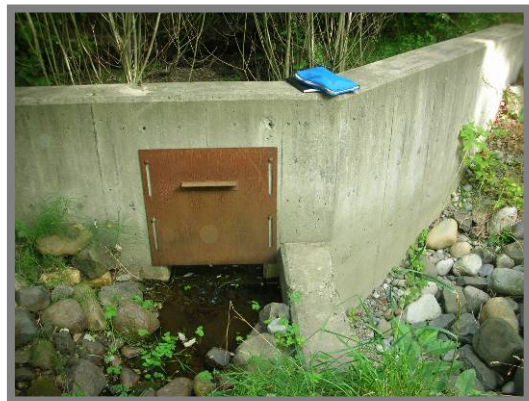
Bifurcation (diversion) structure in Kingfisher Creek
