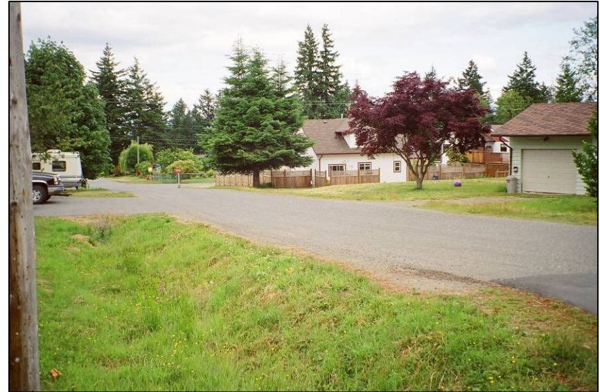
Typical single family residential area, with rural street section; note ditches which could be used as bioswales for runoff treatment
