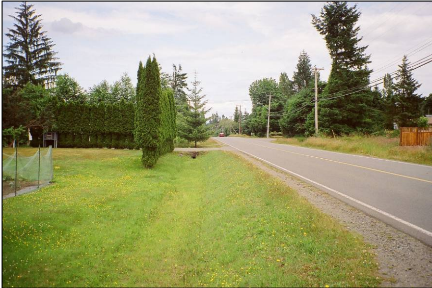
Typical single family residential area, with rural street section; note ditches which could be used as bioswales for runoff treatment
