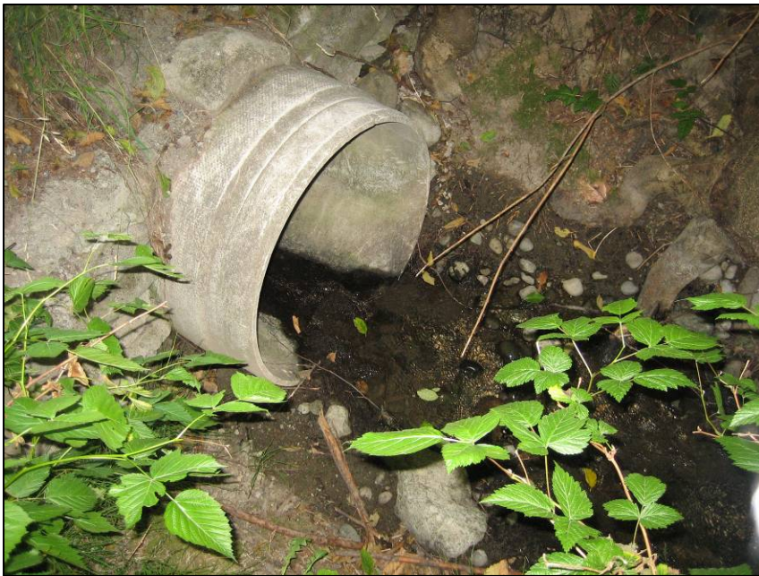
Outlet of 750 mm diameter CMP under Treelane Road; services new development
