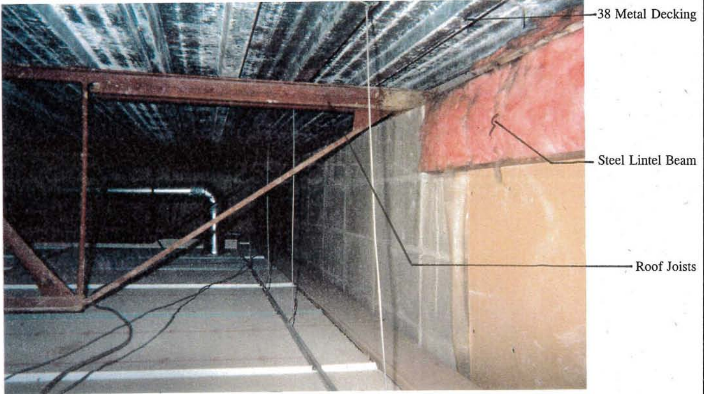
Roof Joist at North Office Wall
