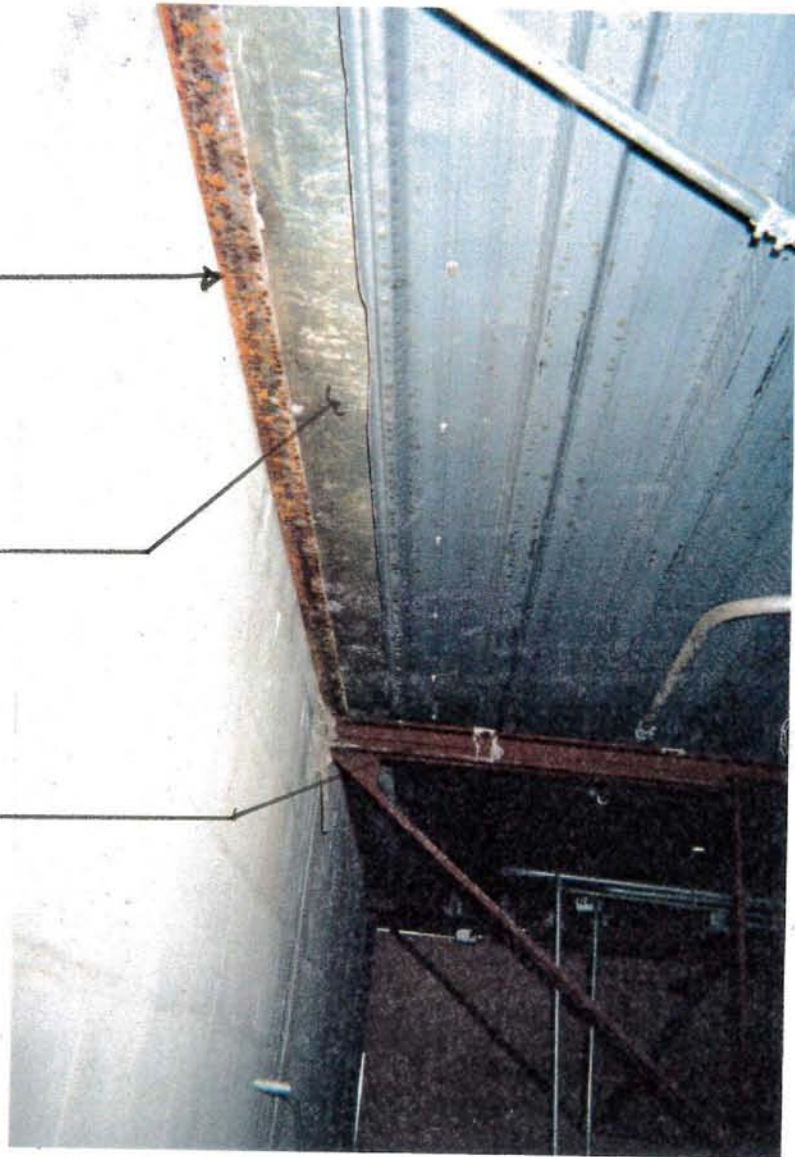
2nd Floor/Masonry Wall Connection Above Locker Room
