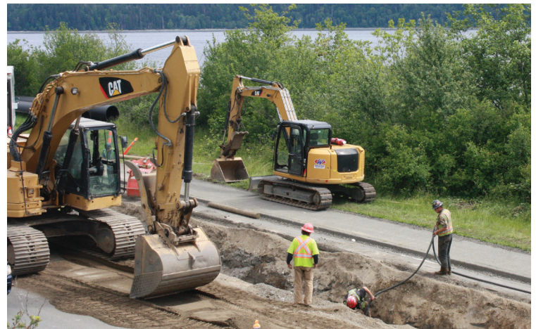
Crews work to install sewer forcemain near the connection point at 1st Ave.
