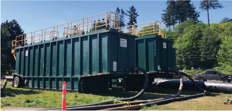
A mobile water treatment system was installed to manage groundwater.
