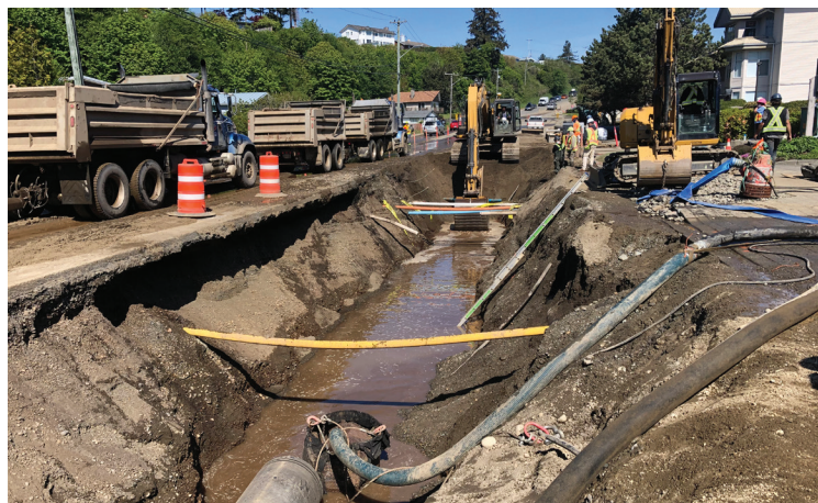
The open trench is prepared for the new sewer pipe to be installed.
