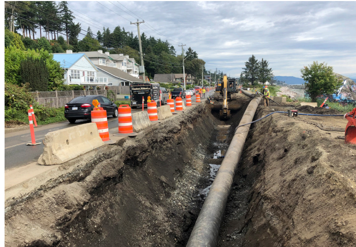
Forcemain installation along Hwy 19A is progressing smoothly.
