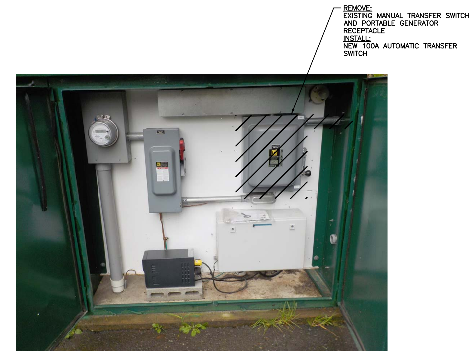
LIFT STATION KIOSK INTERIOR SCALE: N.T.S.
