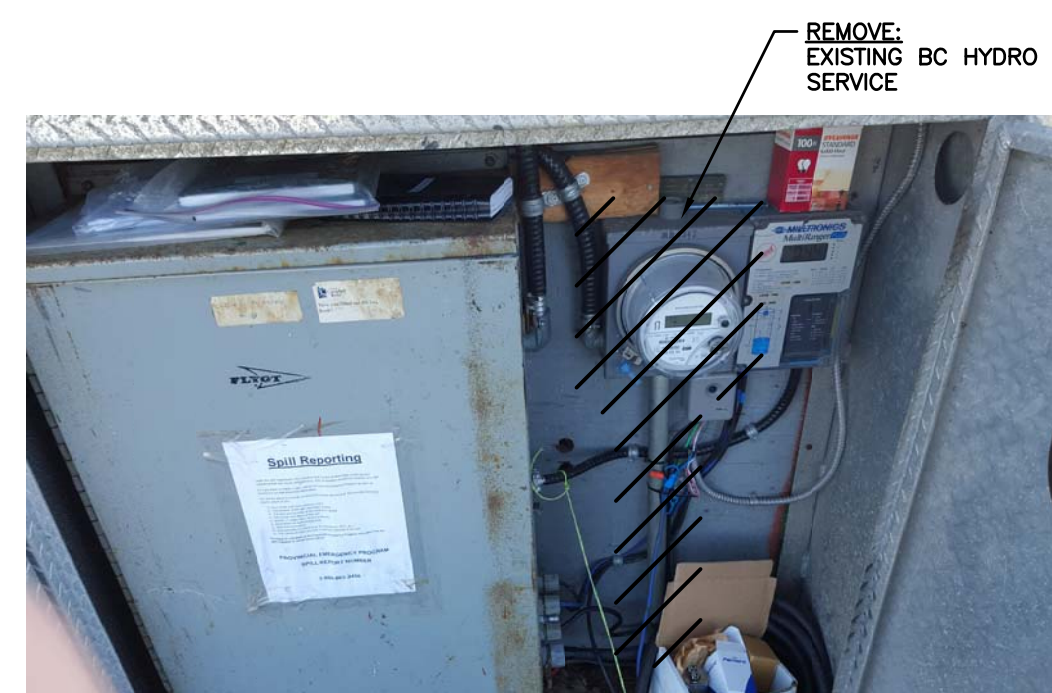
LIFT STATION KIOSK INTERIOR - CONTROL SIDE SCALE: N.T.S.
