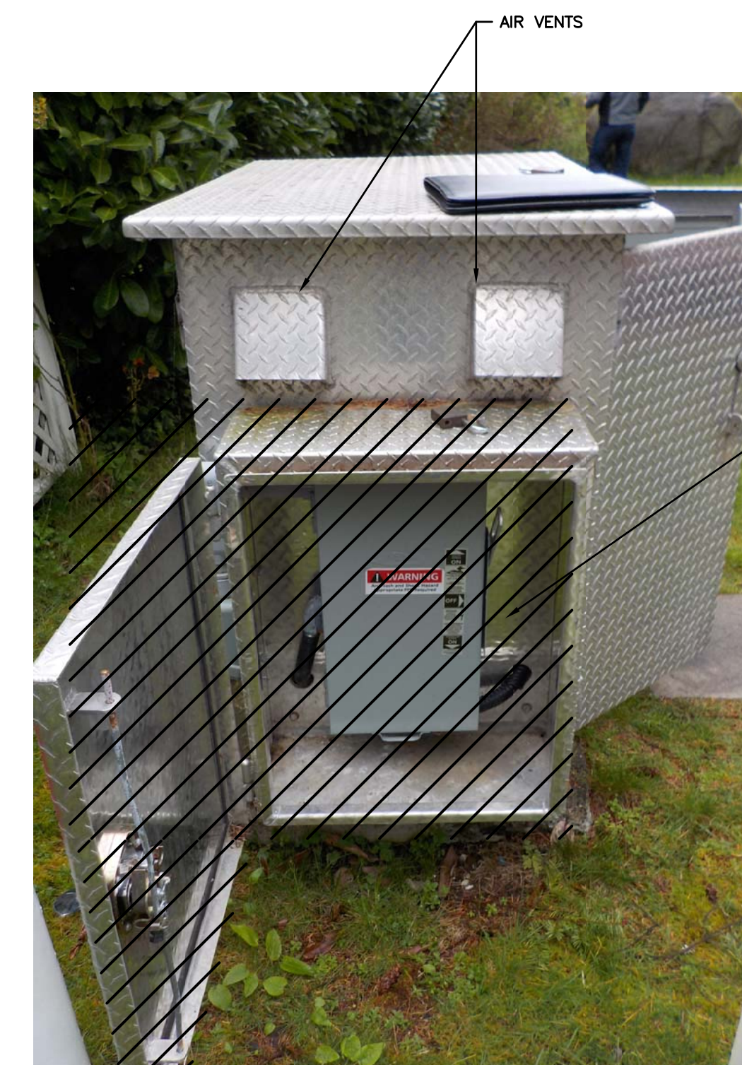
LIFT STATION KIOSK EXTERIOR ENCLOSURE SCALE: N.T.S.
