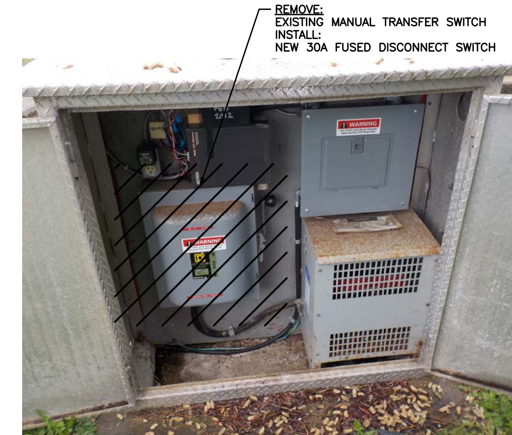
LIFT STATION KIOSK INTERIOR - POWER SIDE SCALE: N.T.S.
