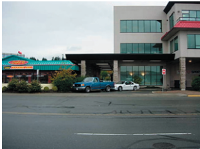
10. Tye Plaza covered walkway
