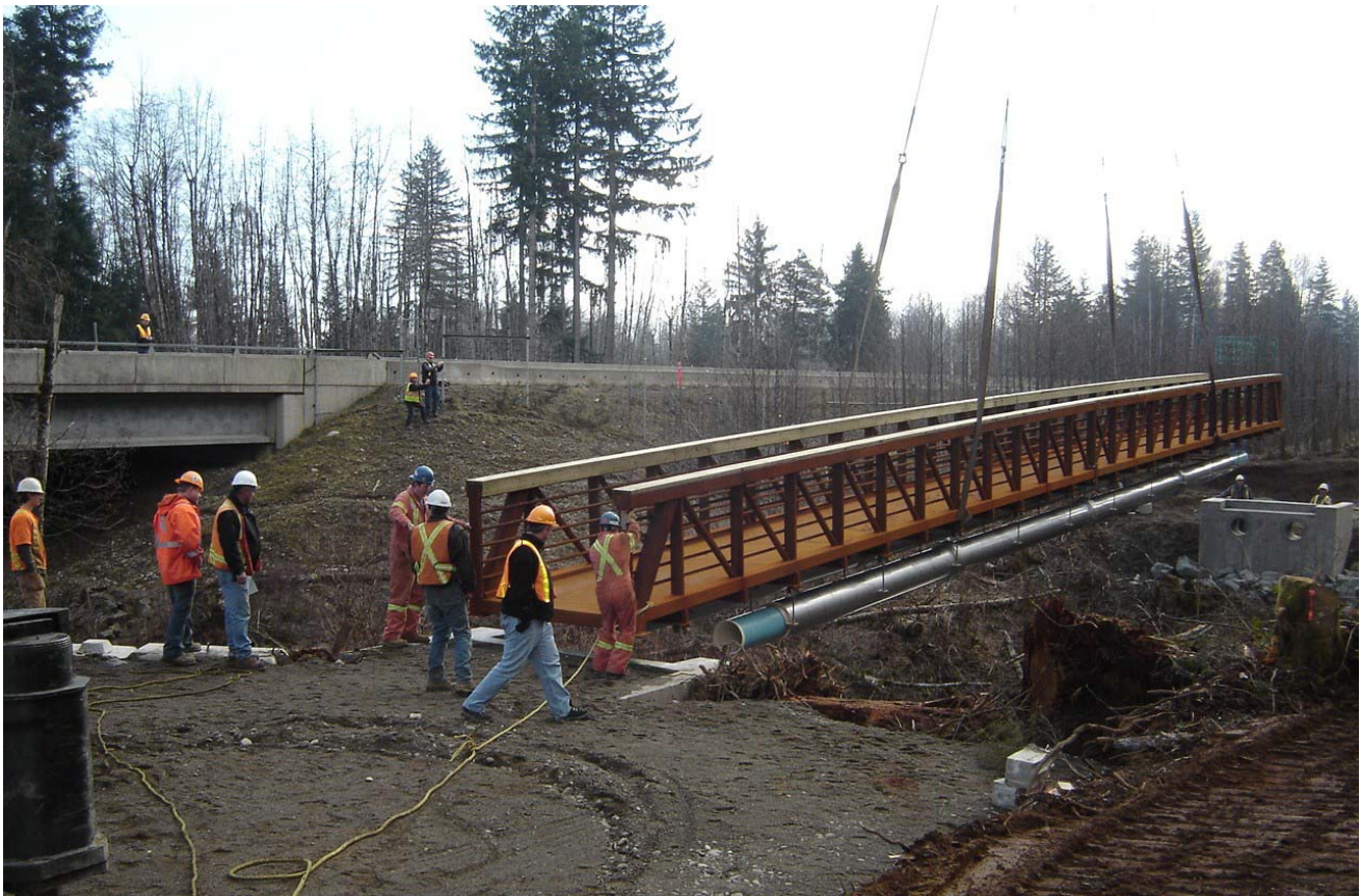
Airport water and sewer main line construction
