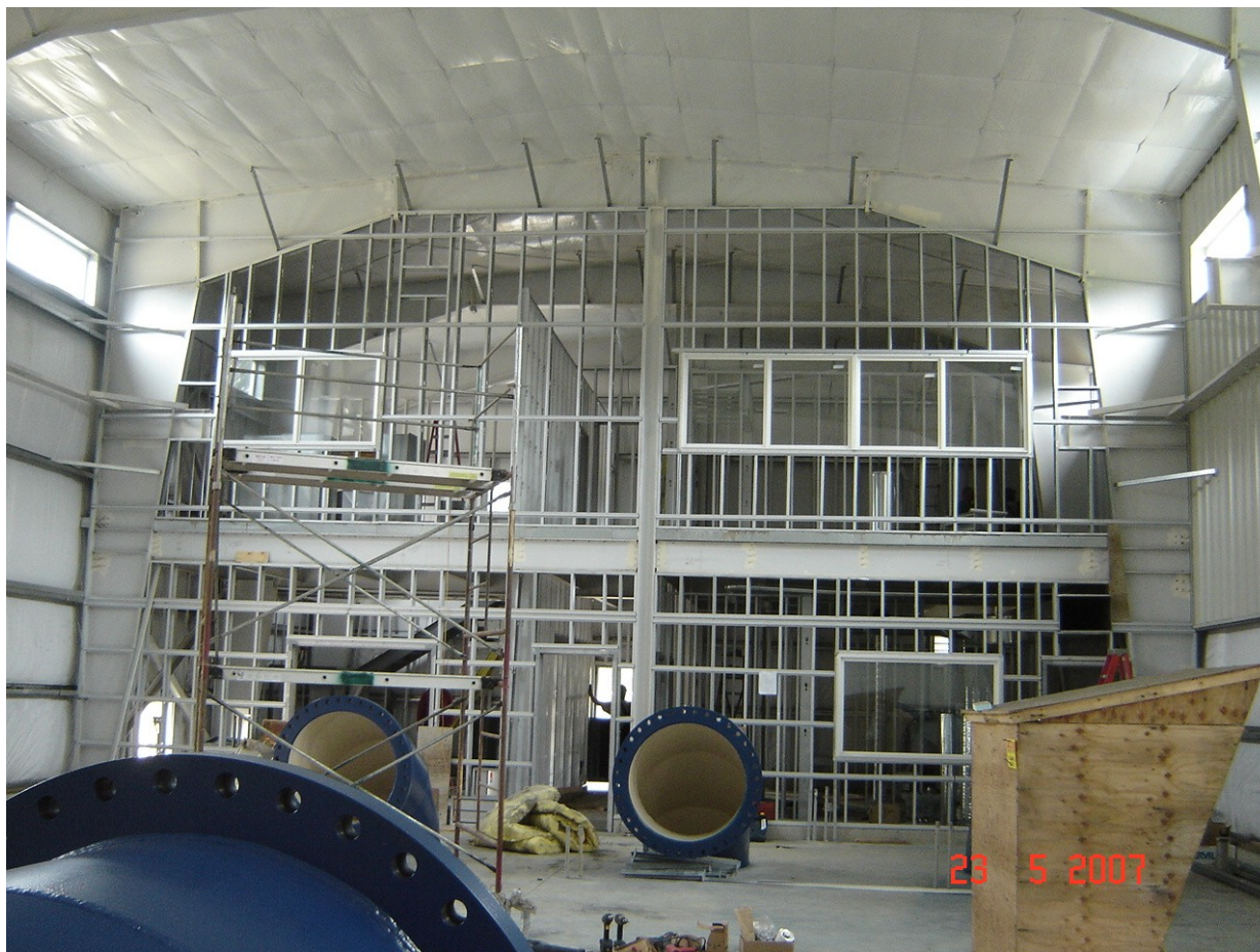
Ultraviolet water treatment facility under construction
