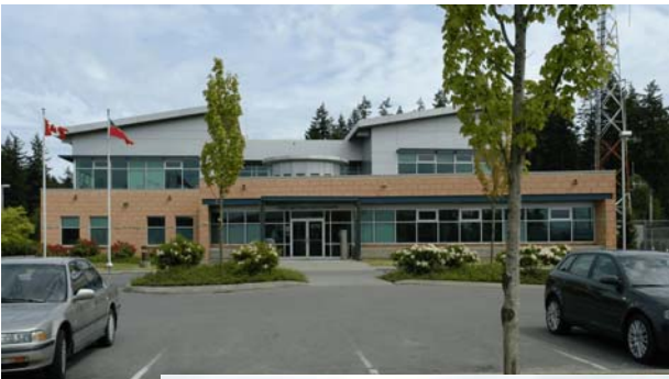
RCMP Detachment Building
