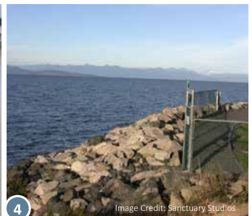
2 Rock armouring replacing seawalls, BC
