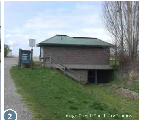
1 Pump station, Netherlands Image Credit: Sanctuary Studios
