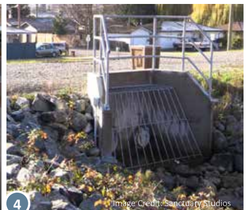
3 Pump station, Netherlands Image Credit: Sanctuary Studios
