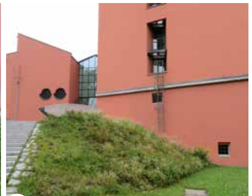
4 Image Credit: Sanctuary Studios Flow-through parking under office, Germany
