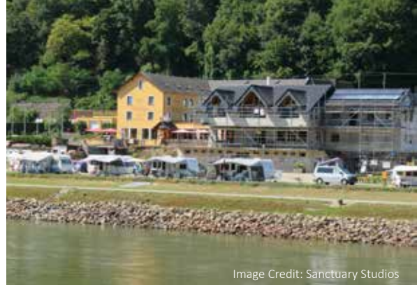
Wet floodproofing and armoring, Germany.
