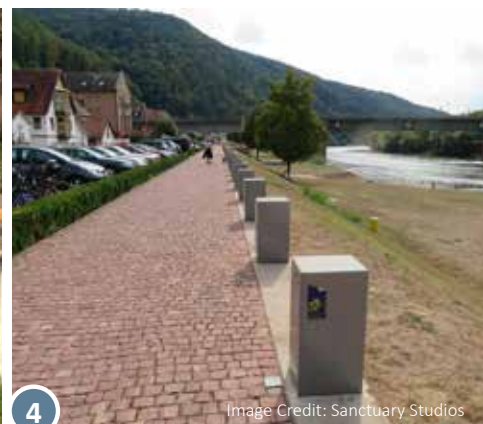
Bollards for temp. flood barrier, Germany
