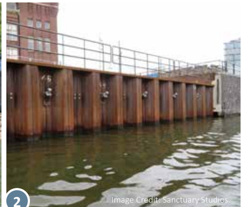
1 Concrete seawall, Austria Image Credit: Sanctuary Studios
