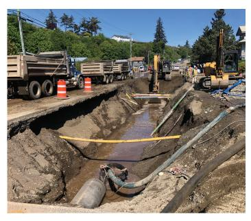
Installing the new waterfront sewer line required deep excavation and careful coordination
