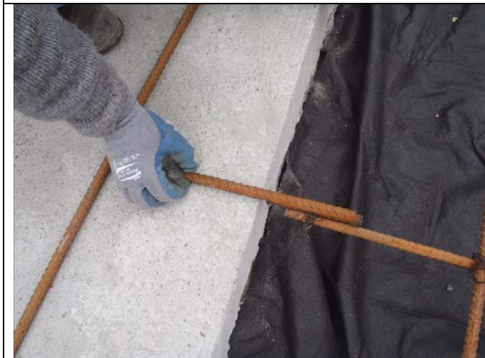
Photo #4: Testing Location #1 Dowel rebar distance into existing cap
