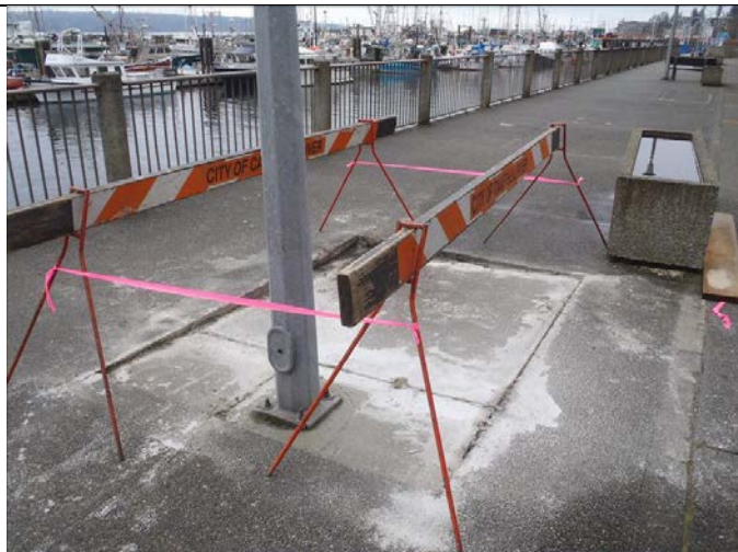
Photo #11: Testing Location #3
