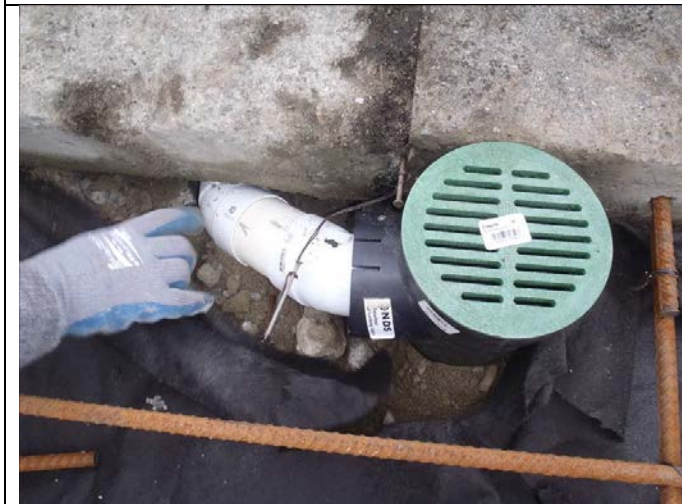
Photo #5: Testing Location #1 Installed drain
