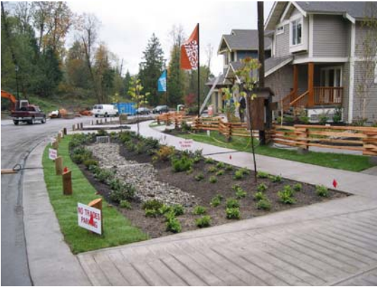
Figure 15: Infiltration Swale (deeper than proposed at Campbell River), Maple Ridge, BC .
