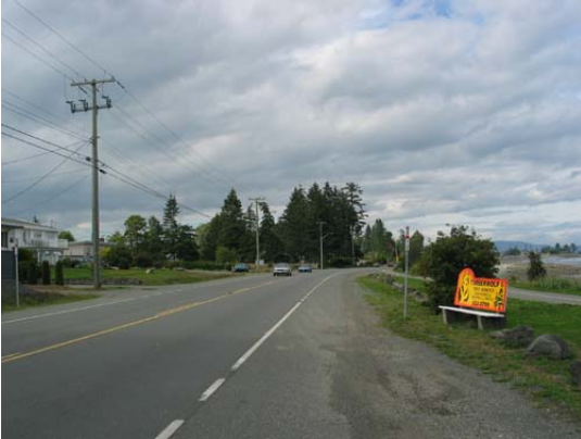
Figure 2: Existing South Island Highway in Campbell River .
