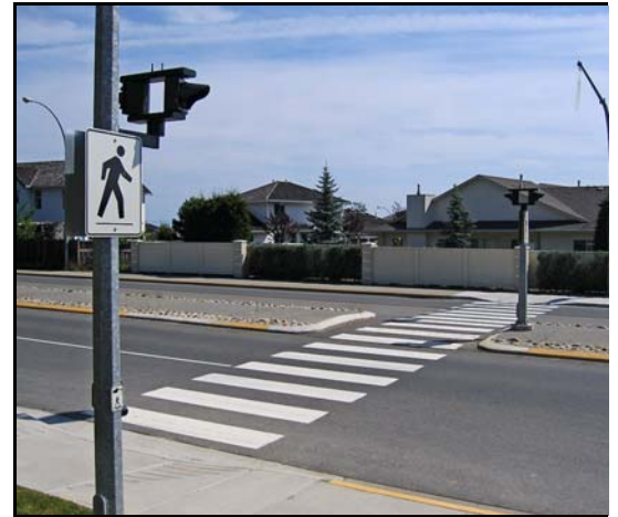
Figure 10 — Flashing lights at crosswalk, Nanaimo .
